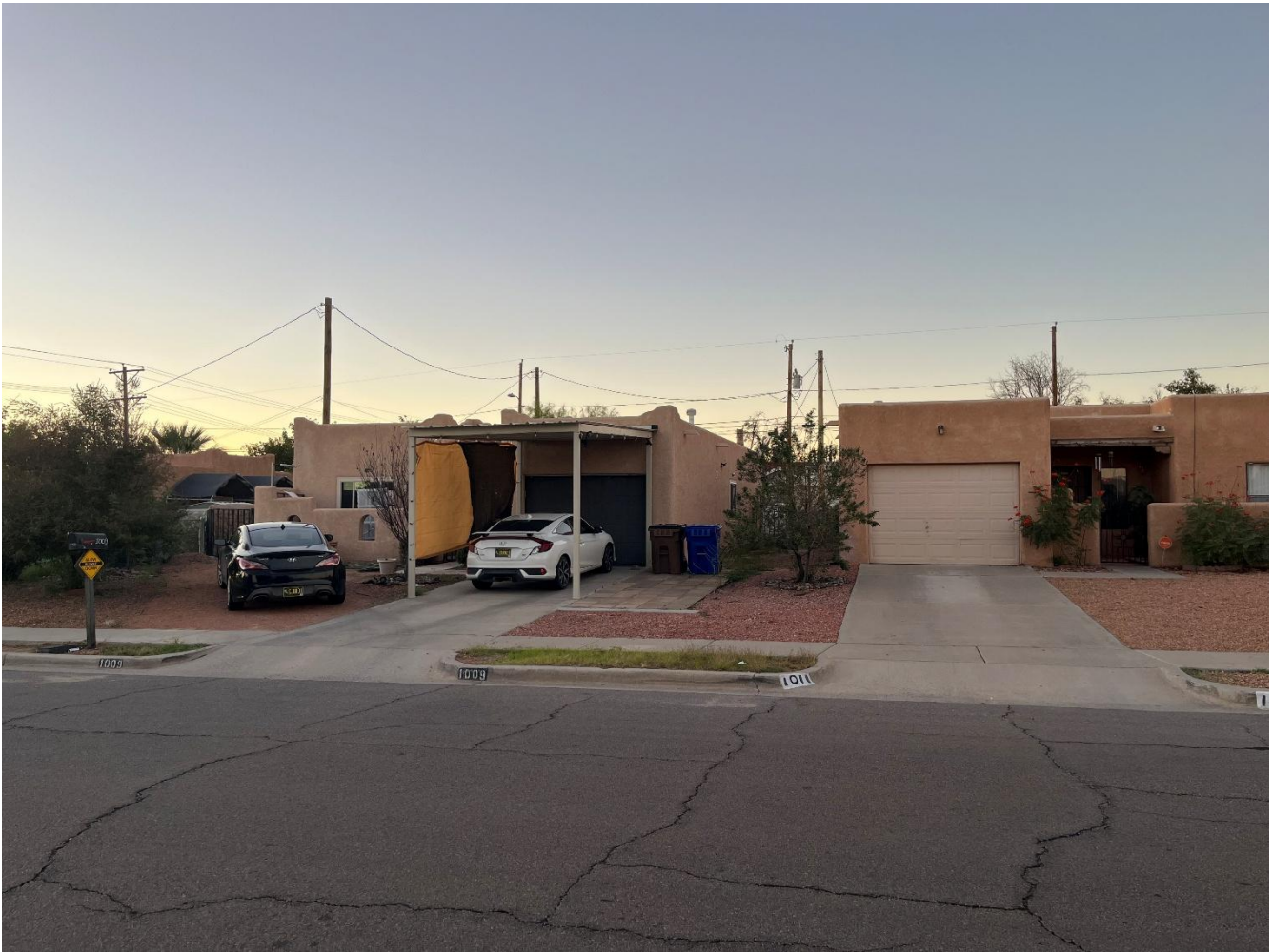
Figure 3: The carport at 1009 E. Court Avenue.
