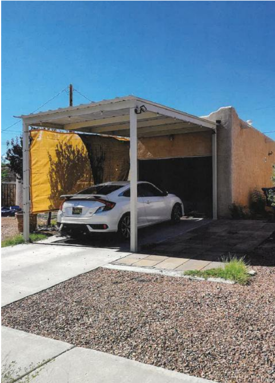
Figure 5: Photograph of the carport, courtesy of the property owner.
