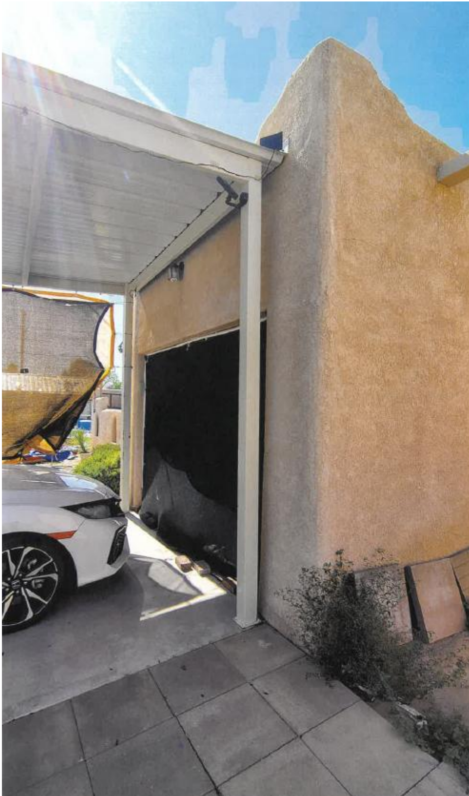
Figure 6: Photograph of the front detail of the carport, showing its attachment to the residence, courtesy of the property owner.
