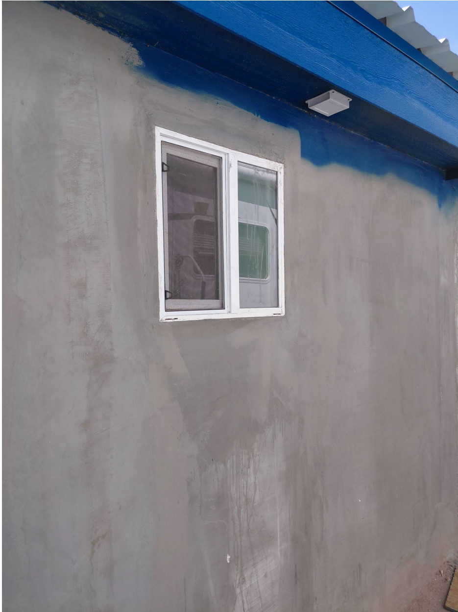
Figure 12: Former location of side door, now small slider.
