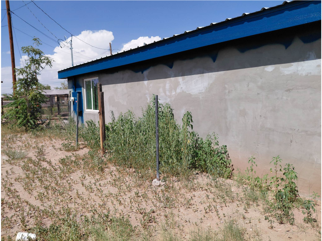
Figure 16: Slider on north side of west façade; two windows have been removed.
