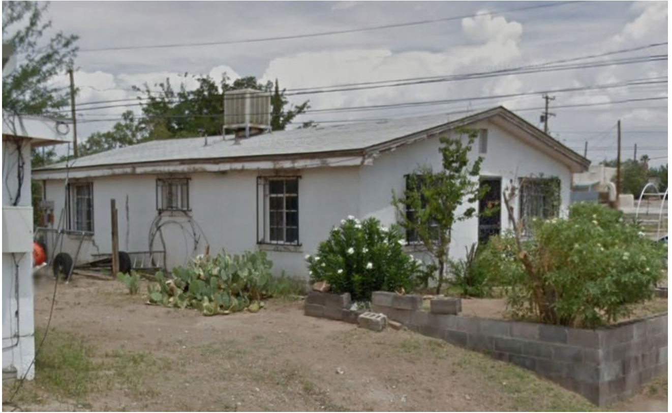
Figure 4: Google Streetview screenshot of house. 2011, showing windows on the west façade.
