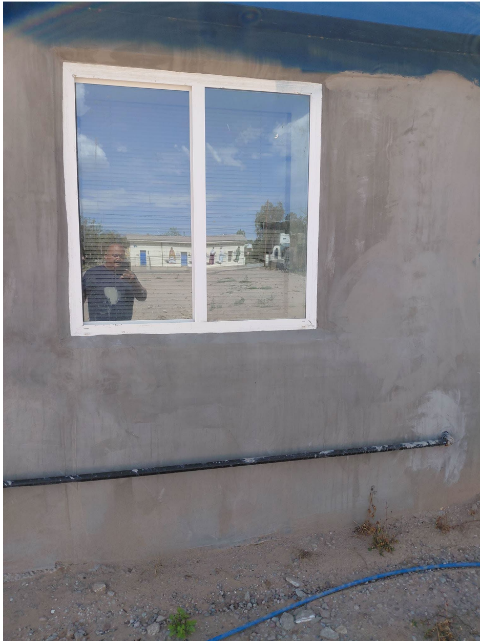
Figure 10: Window closest to front of building on east façade, formerly a steel casement window.
