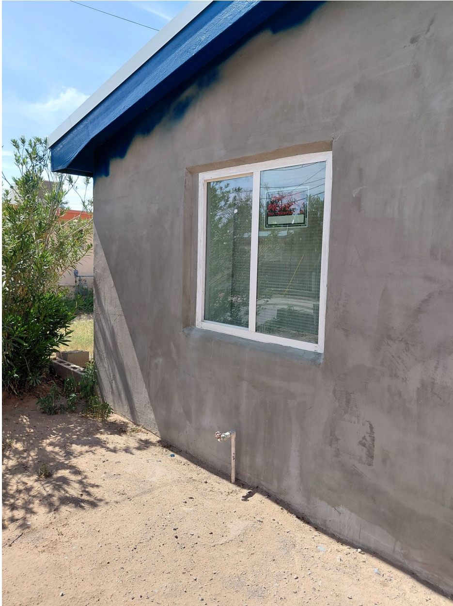
Figure 7: Replacement window on front façade, to the left of the front door.
