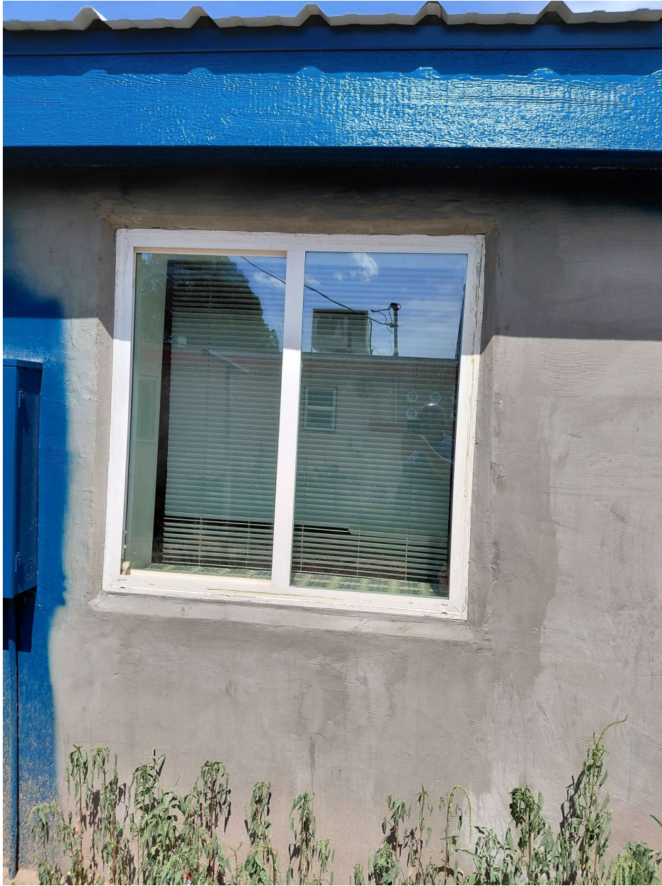
Figure 17: New window on west façade.
