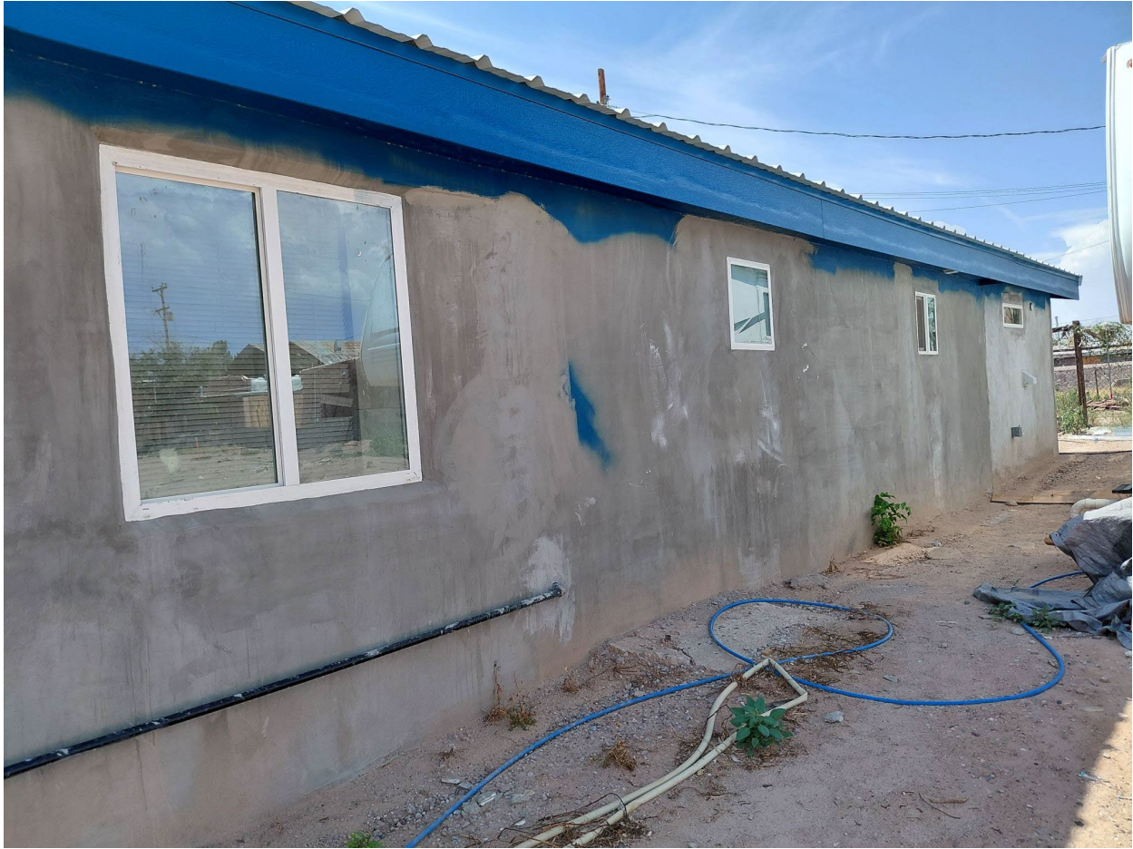
Figure 9: East façade of property, showing new windows, including removal of side doorway and addition to the rear.
