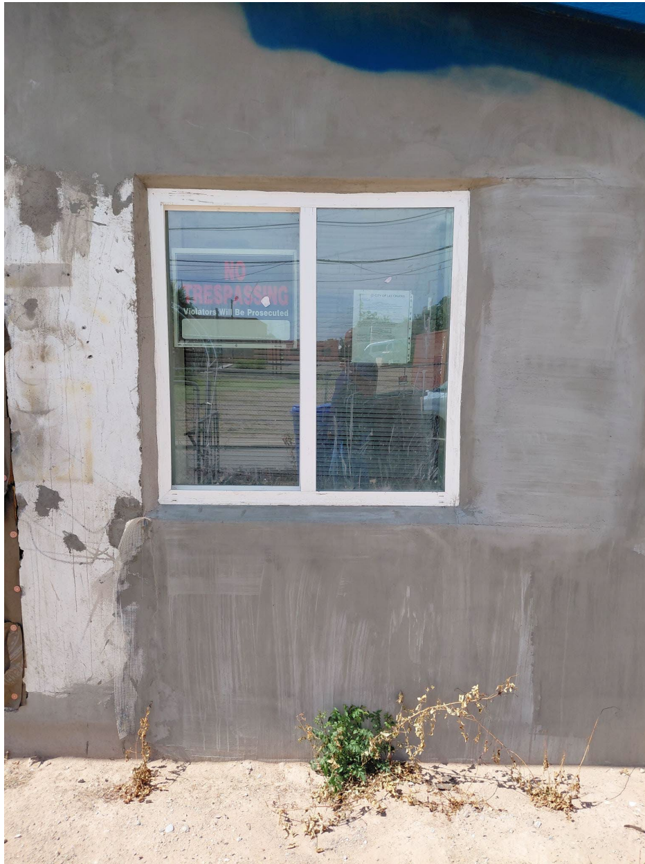
Figure 8: Replacement window on front façade, to the right of the front door.
