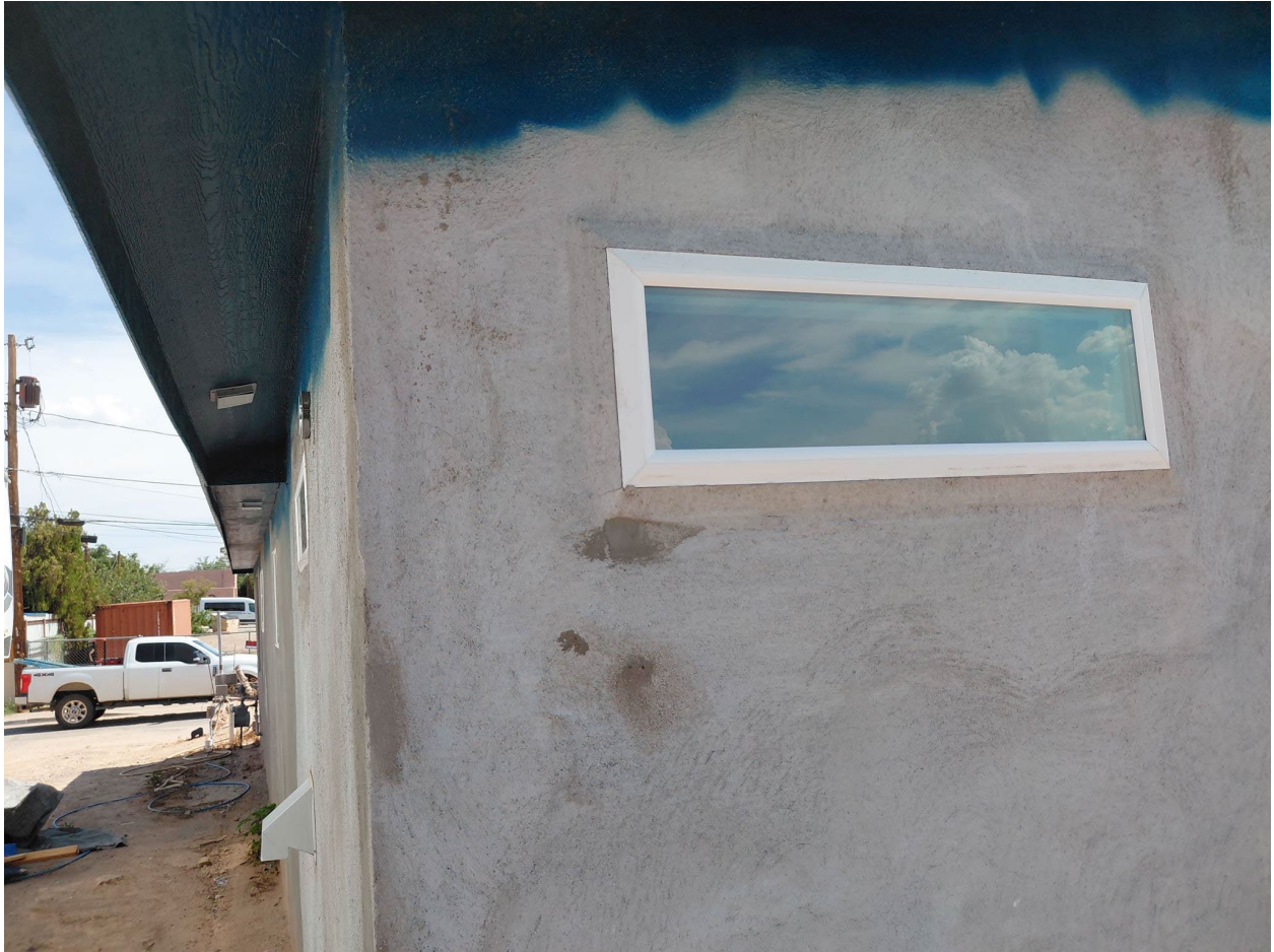
Figure 14: Clerestory window on north façade of addition.
