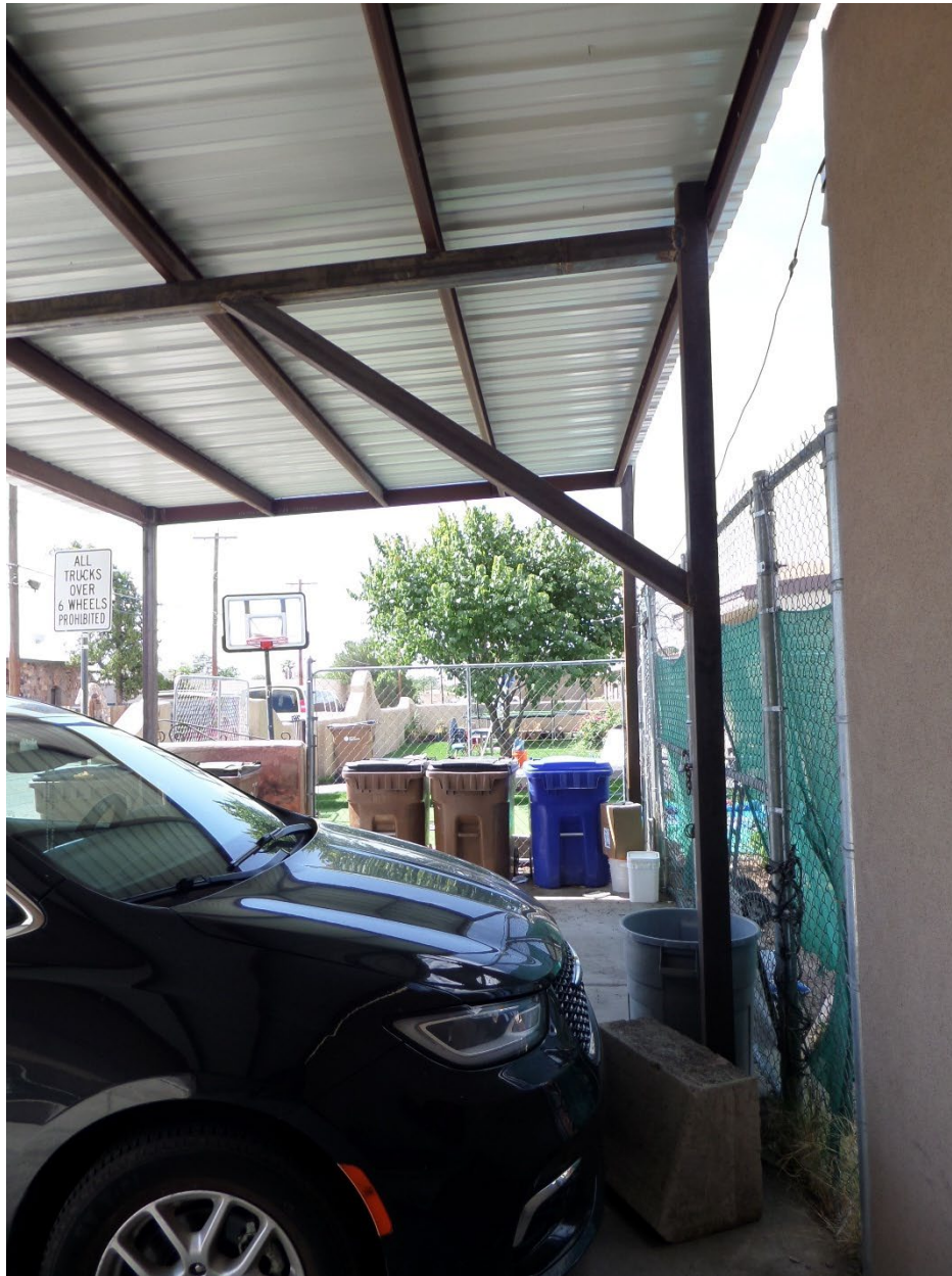
Figure 8: Central post on the west side of the carport, supported by a knee brace.
