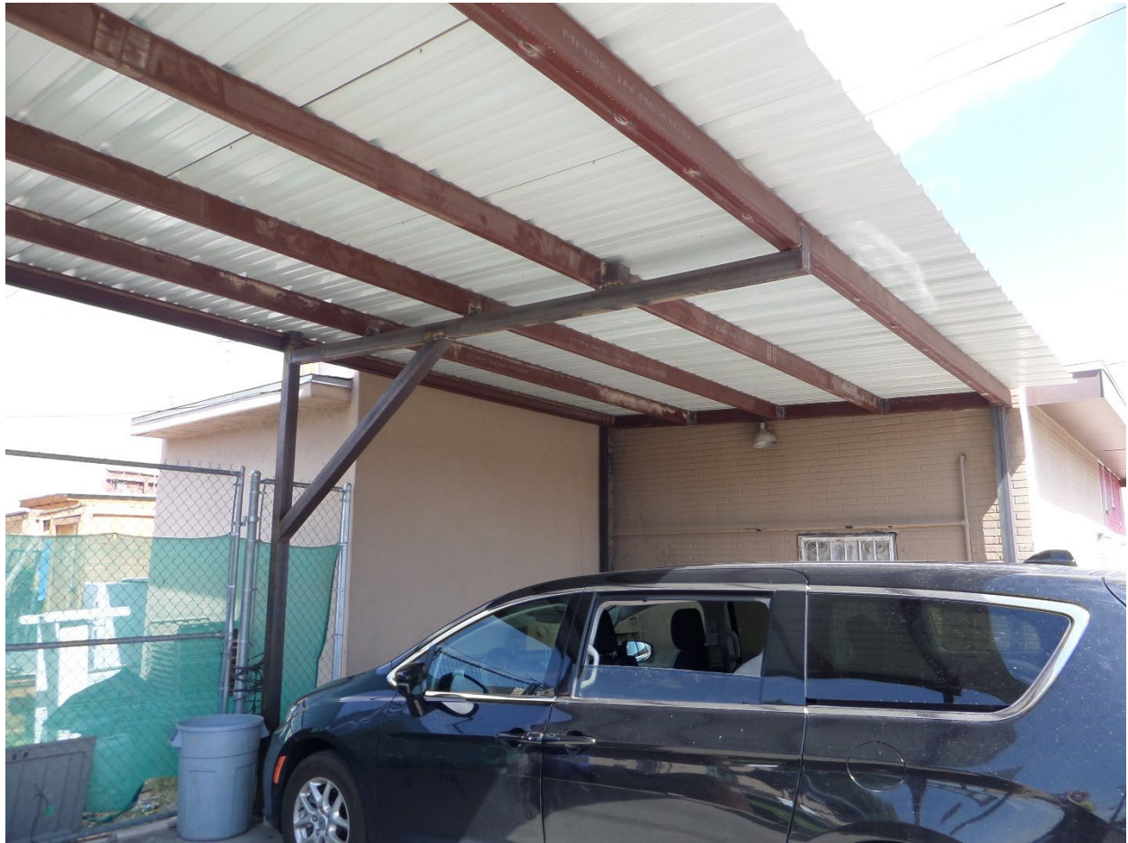
Figure 5: Detail of the carport where it meets the building. While the carport does not appear to be directly fixed to the bakery building, it's placement is close enough to describe it as an addition to the main building; the two roofs will also work in tandem when shedding water, meaning the carport will become an extension of the building system.
