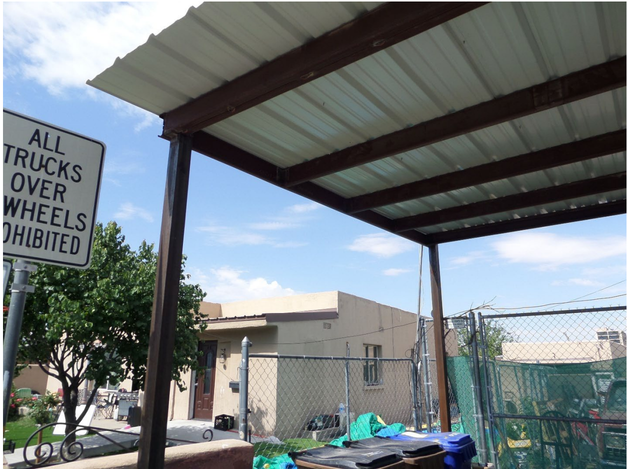
Figure 4: Detail of the carport construction.
