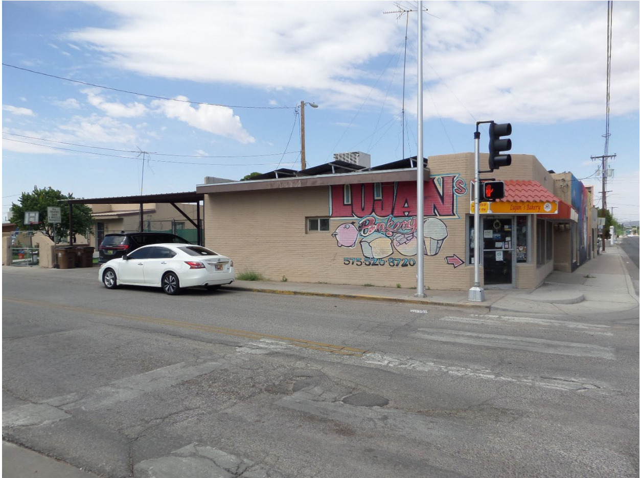
Figure 2: Lujan Bakery at 442 N. Lohman Avenue, carport to the rear (south) of the main building.
