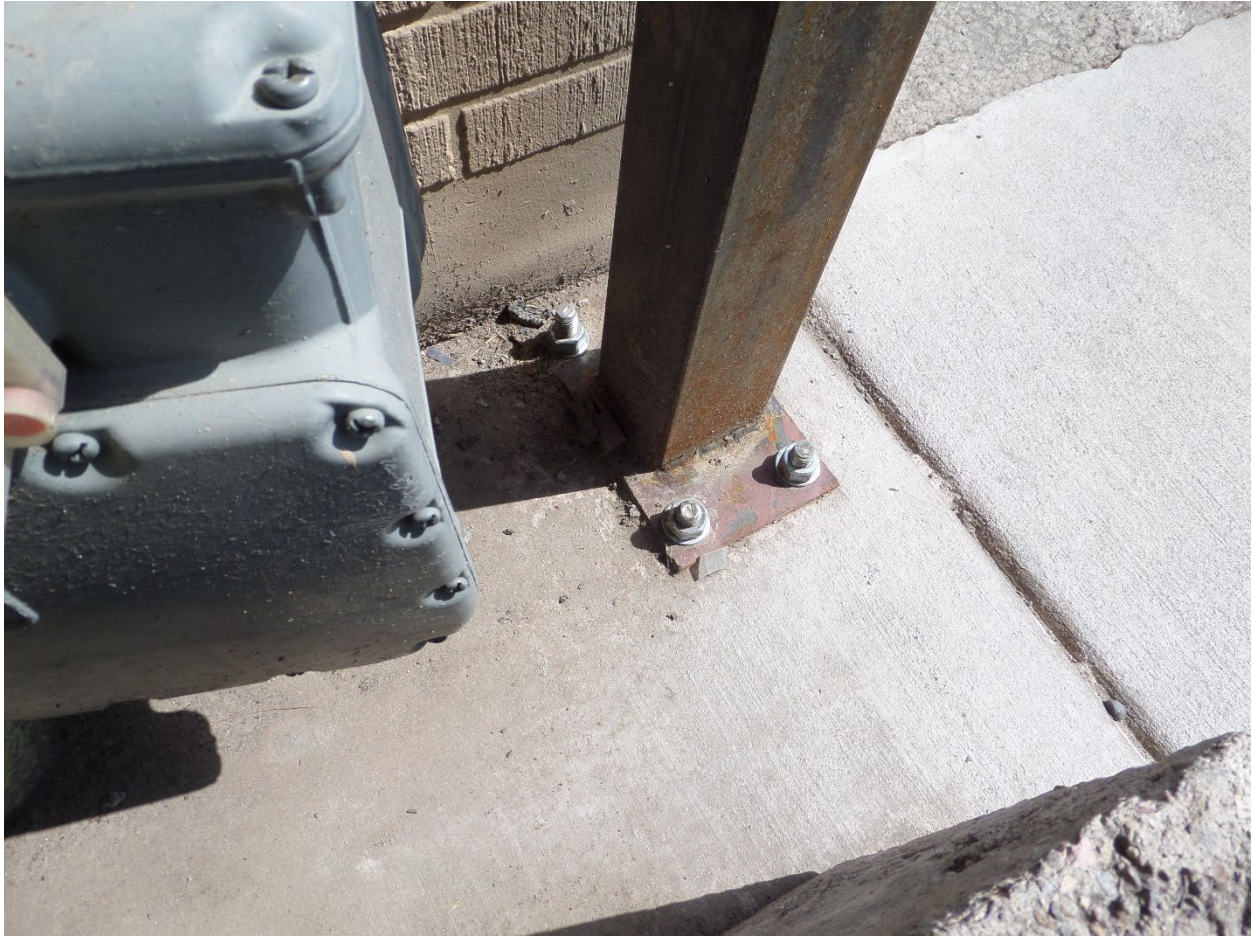
Figure 6: An example of the carport's post footer with base plate and anchor bolts on top of a concrete pad.
