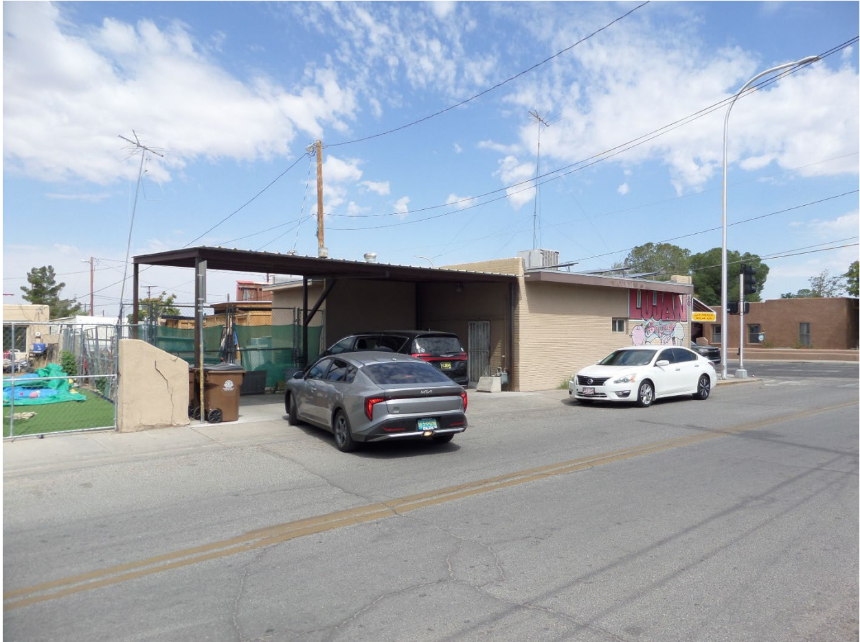
Figure 3: Carport to the rear (south) of the main building. The carport mirrors the roof-plane of the bakery building and is not higher than the surrounding buildings.
