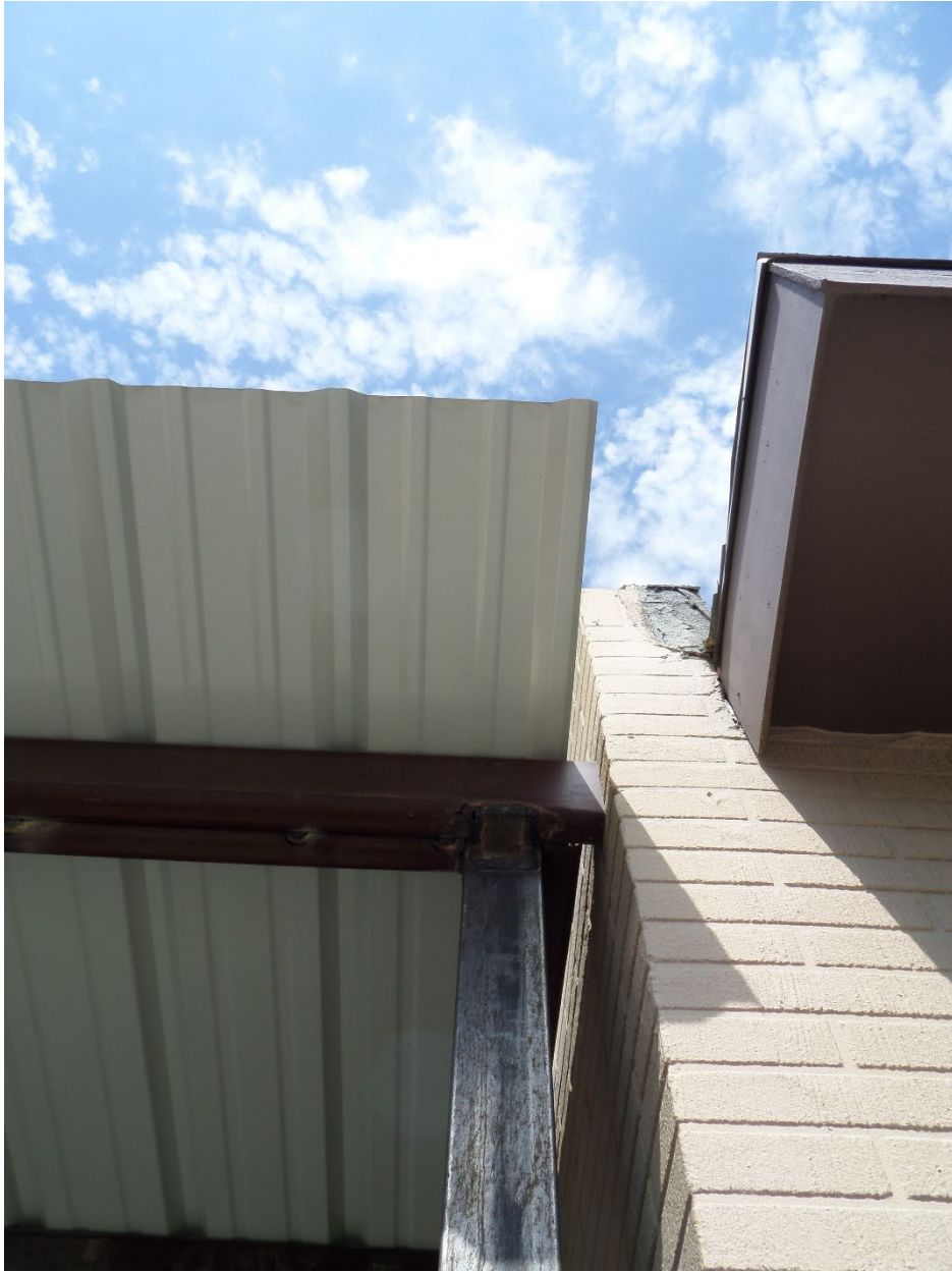
Figure 7: Carport against the bakery building.
