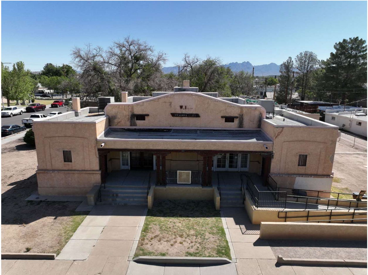
Figure 6: Aerial photo of the WIA building, showing the accessibility ramp to the right.
