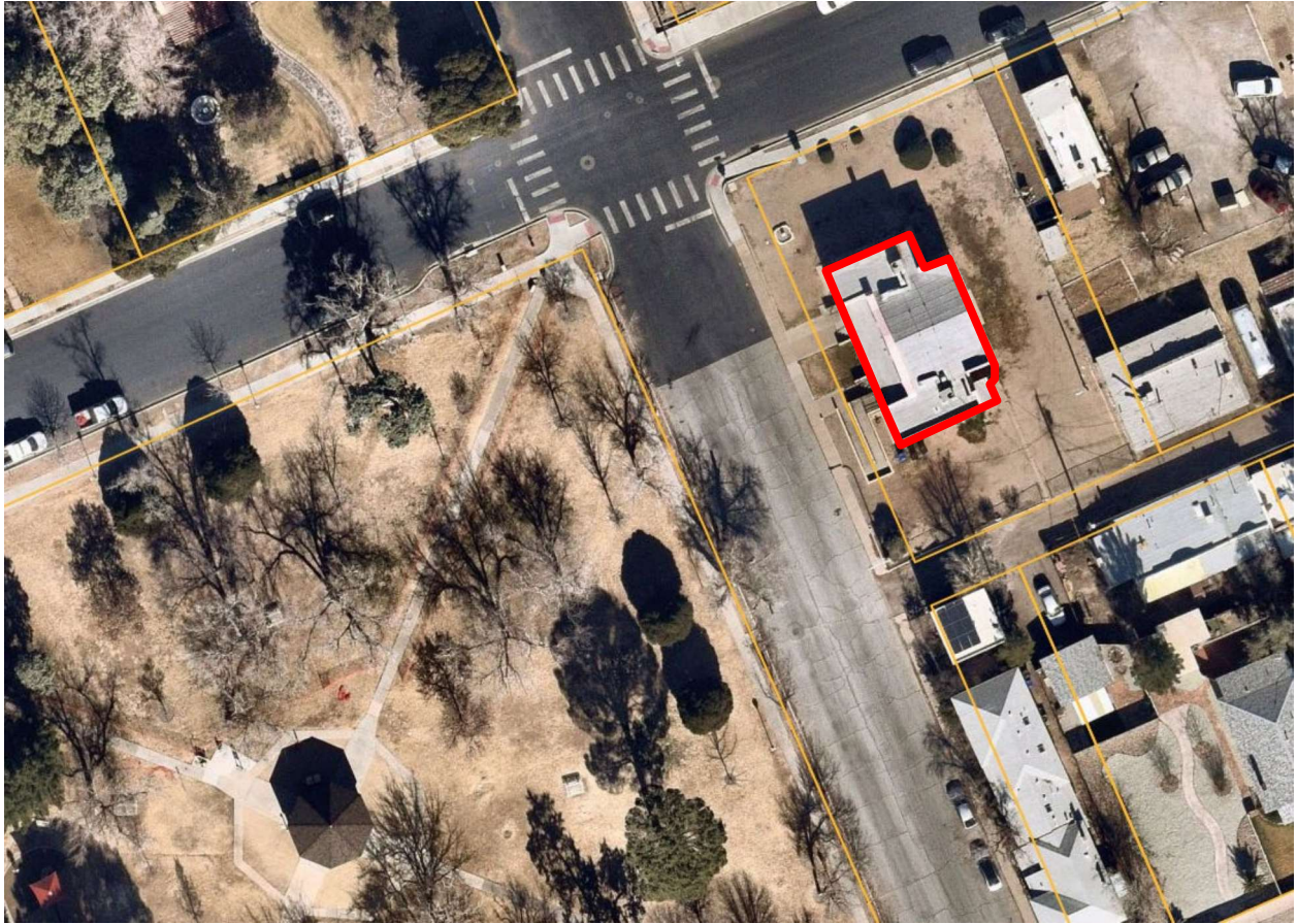
Figure 1: WIA property at 340 N. Raymond Street; building is highlighted in red.
