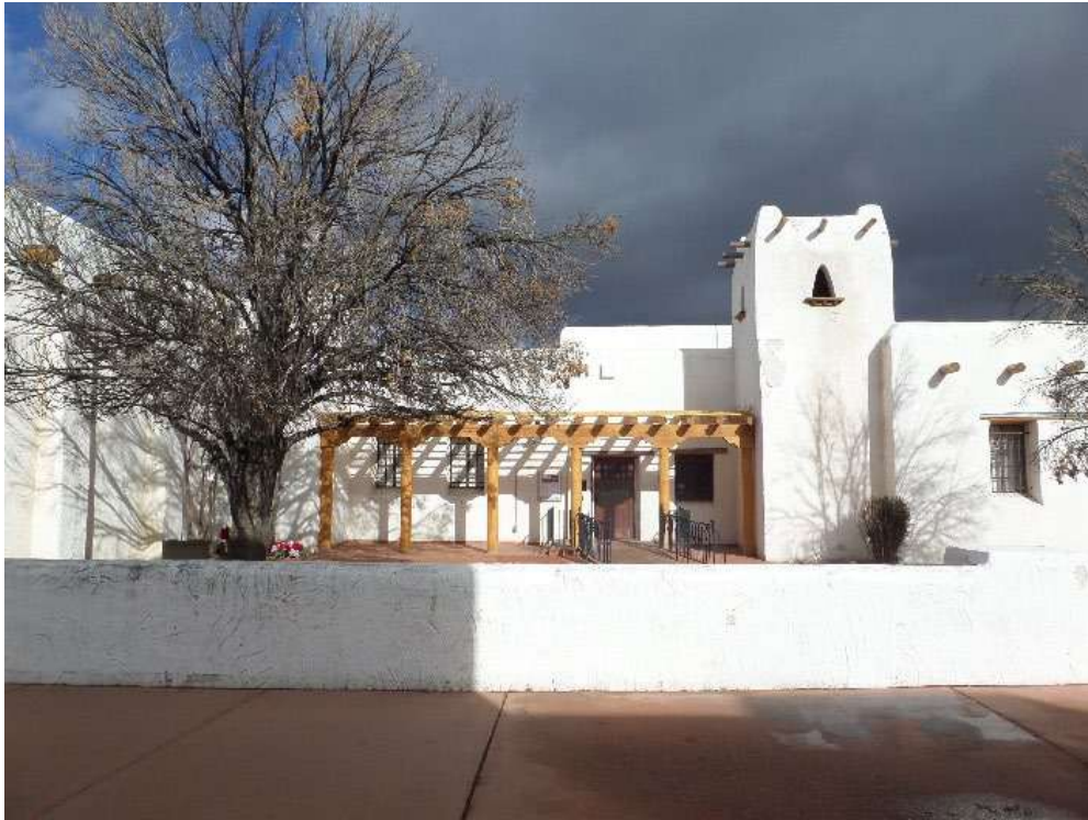
Figure 1: Front of building, facing north.
