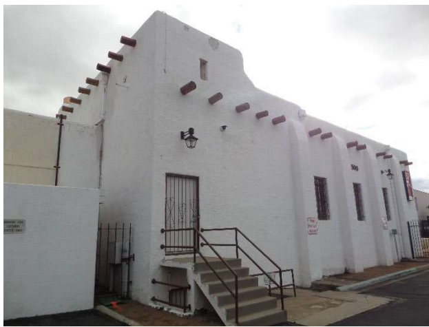
Figure 4: West façade of the building, service entrance behind the stage in the former auditorium.
