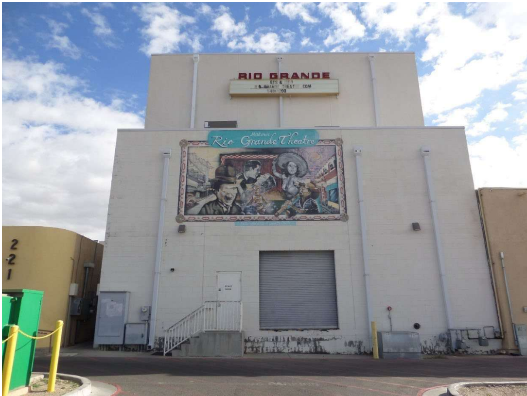
Figure 4: Rear of building, showing loading dock and back entrance.
