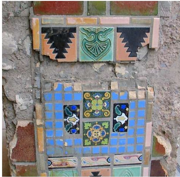
Figure 15: Photograph of the uncovered tiles on the front of the building, prior to restoration in the 2000s. Photo credit, Las Cruces Blog – News, Photos, History “Rio Grande Theatre” post, October 16, 2007.
