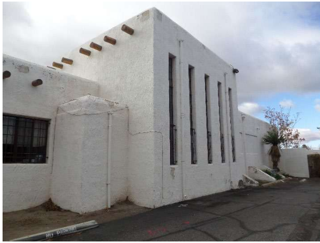
Figure 3: Rear of the building, facing south.
