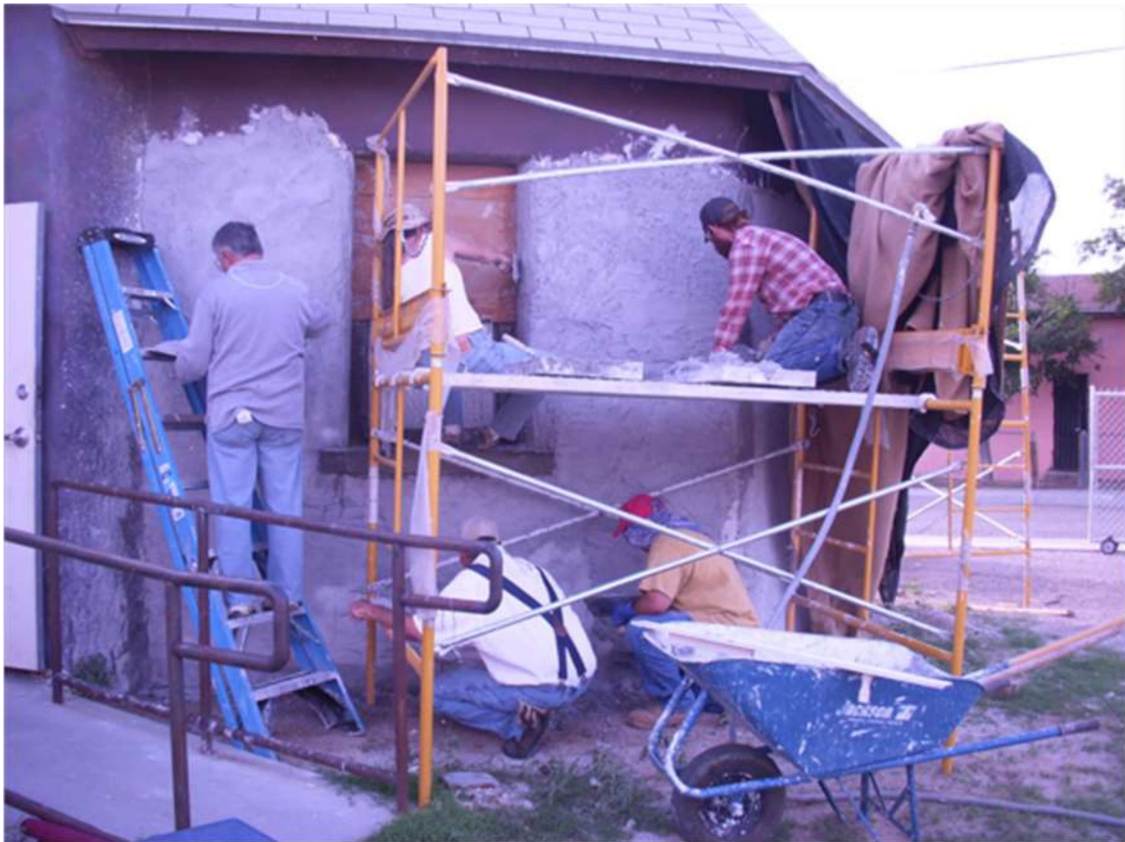
Figure 42: Applying another application of scratch coat lime plaster to the apse, 2012. Left on ladder David Chavez. On top of scaffolding L - R: Faith Hutson and Dan Carter. Bottom of scaffolding L-R: John Hyndman and Dominic Fiumara. (Courtesy of Faith Hutson).
