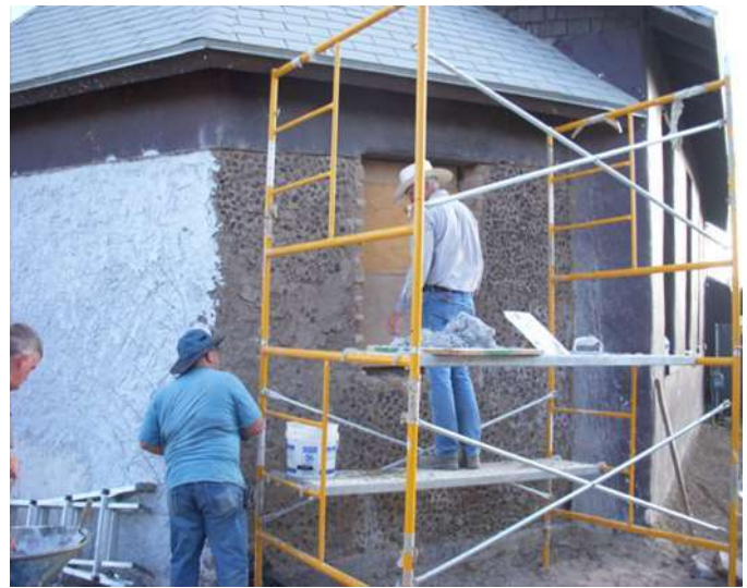
Figure 27: Apse wall repair Summer 2010. Pat Taylor is on the scaffolding, Dominic Fiumara is to the left. (Courtesy of Faith Hutson).
