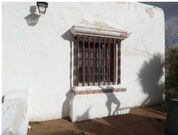
Figure 7: Southwest corner of the building, featuring a distinct window decorated with extended hood and sill, supported by ornamented wooden doweling.
