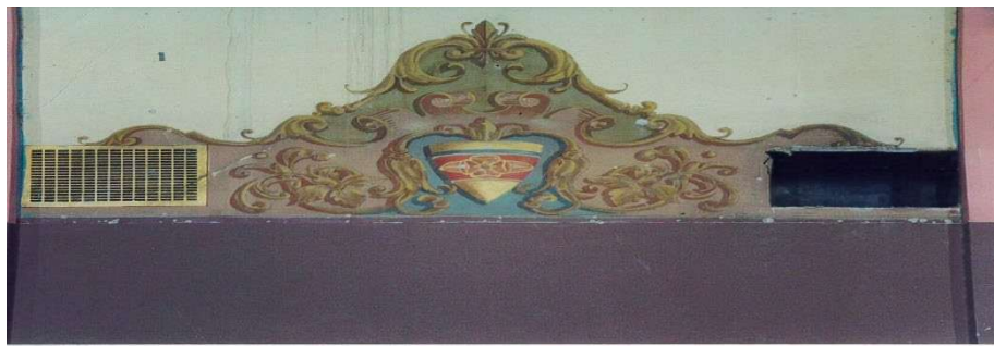
Figure 16: Original scrollwork and cooling system ducts on the interior of the theatre, taken in 1998 as part of the restoration.
