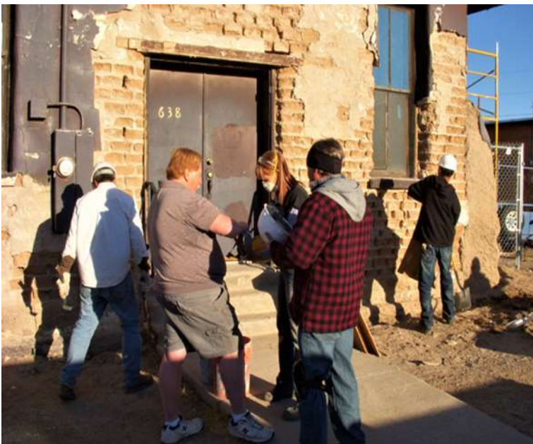
Figure 35: Removal of cement stucco on the front of the church, February 2011. Instructor Keven Gall, left with students. (Courtesy of Faith Hutson).
