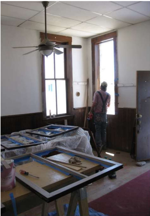
Figure 43: John Hyndman working on window restoration, 2012. (Courtesy of Faith Hutson).
