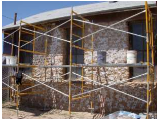
Figure 25: Application of rajuelas on the south side wall April 2010. (Courtesy of Faith Hutson).
