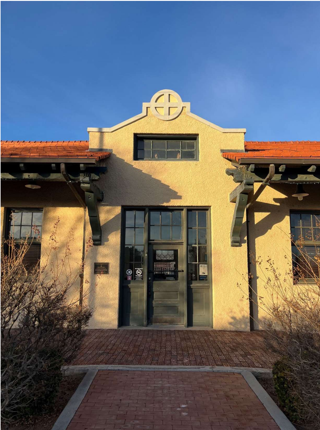
Figure 3: Photo of the main entrance to the depot, with the high clerestory window visible just below the AT&SF symbol in the extruded dormer.
