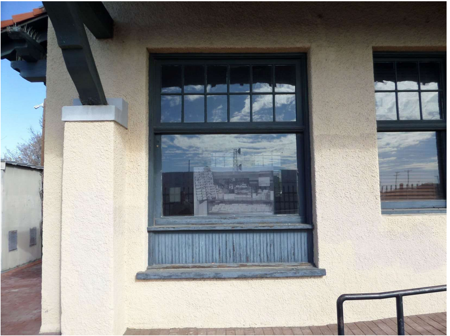
Figure 7: The single-hung window for the station's newsstand, with a matching lite configuration on top of the movable frame.
