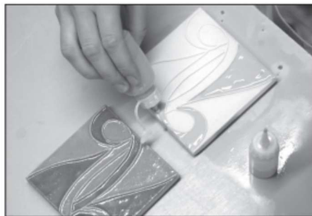
Tiles found in a crawl space of a San Jose, Calif., home have become the basis for the tile restoration plan.
