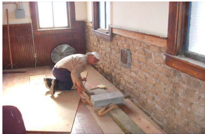
Figure 29: North Wall repair by Fred Apodaca Summer 2010. (Courtesy of Faith Hutson).
