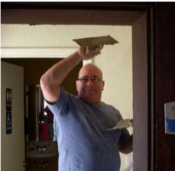
Figure 45: Interior plaster repair by Dominic Fiumara, 2013. (Courtesy of Faith Hutson).
