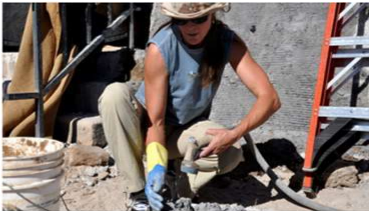
Figure 39: Faith Hutson mixing lime for a scratch coat application, 2011. (Courtesy of Darla Matthew).
