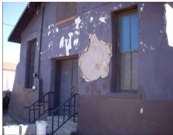
Figure 21: West side entrance, February 2010. (Courtesy of Faith Hutson).
