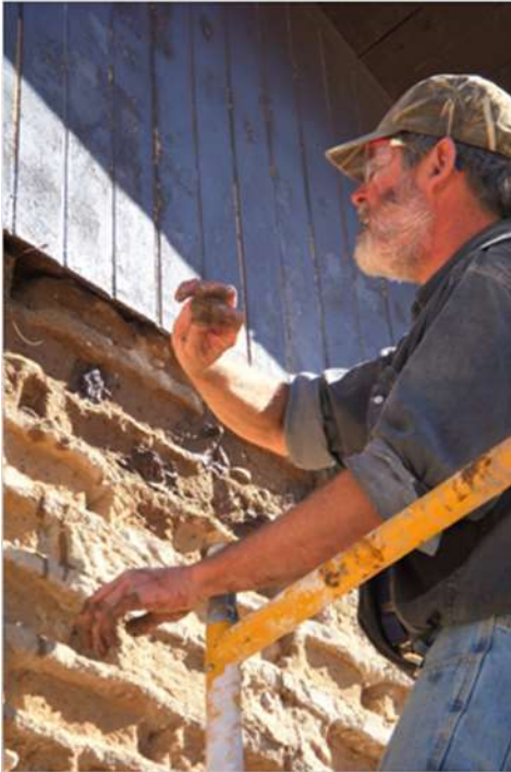
Figure 37: John Hyndman applies mud mortar to set rajuelas, 2011. (Courtesy of Faith Hutson).
