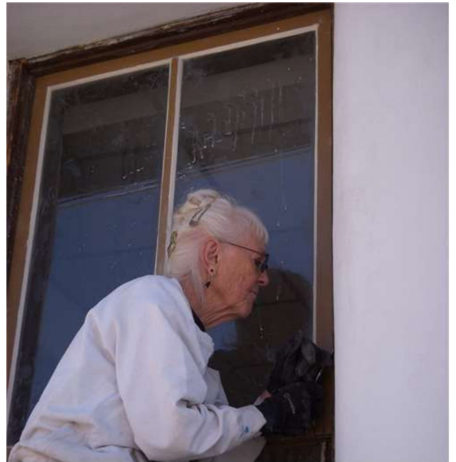
Figure 44: Wilma Hutson scraping old paint from window frames, 2012. (Courtesy of Faith Hutson).
