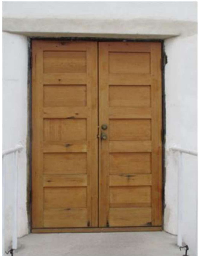
Figure 49: Replica doors made by Watson McKennon, 2014. (Courtesy of Beth O'Leary).
