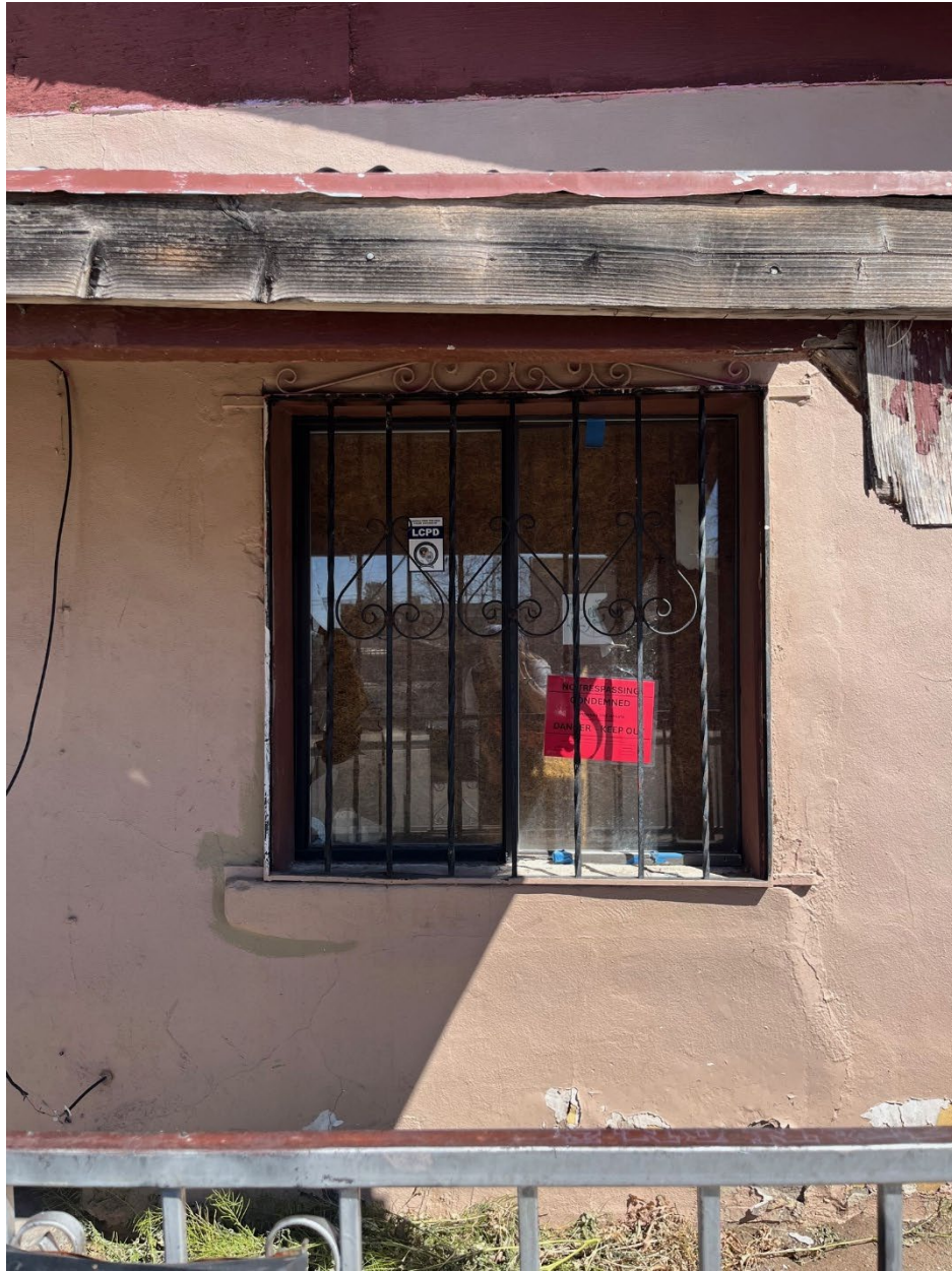
Figure 4: South window on main façade of the house fronting San Pedro Street.
