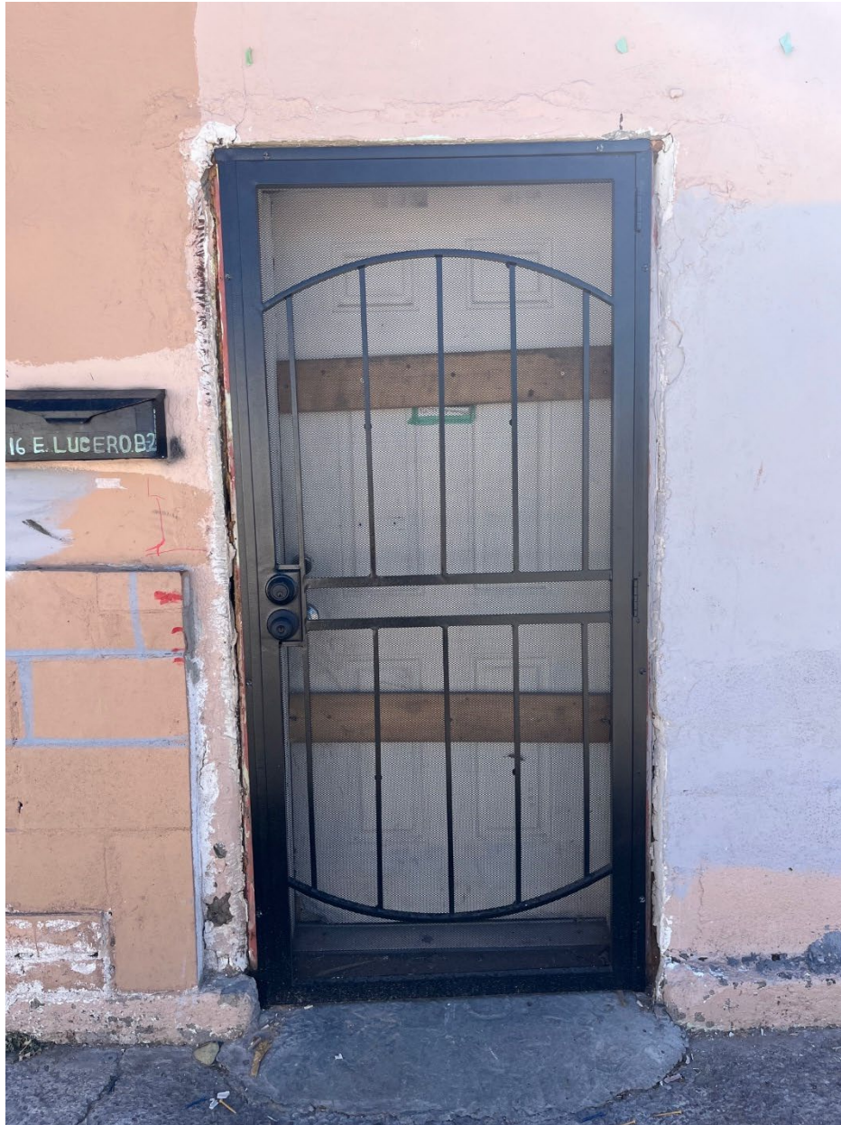
Figure 8: Door on west unit of the duplex on Lucero Avenue.
