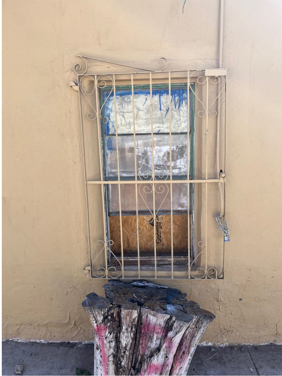
Figure 12: Window on east unit of the duplex on Lucero Avenue.
