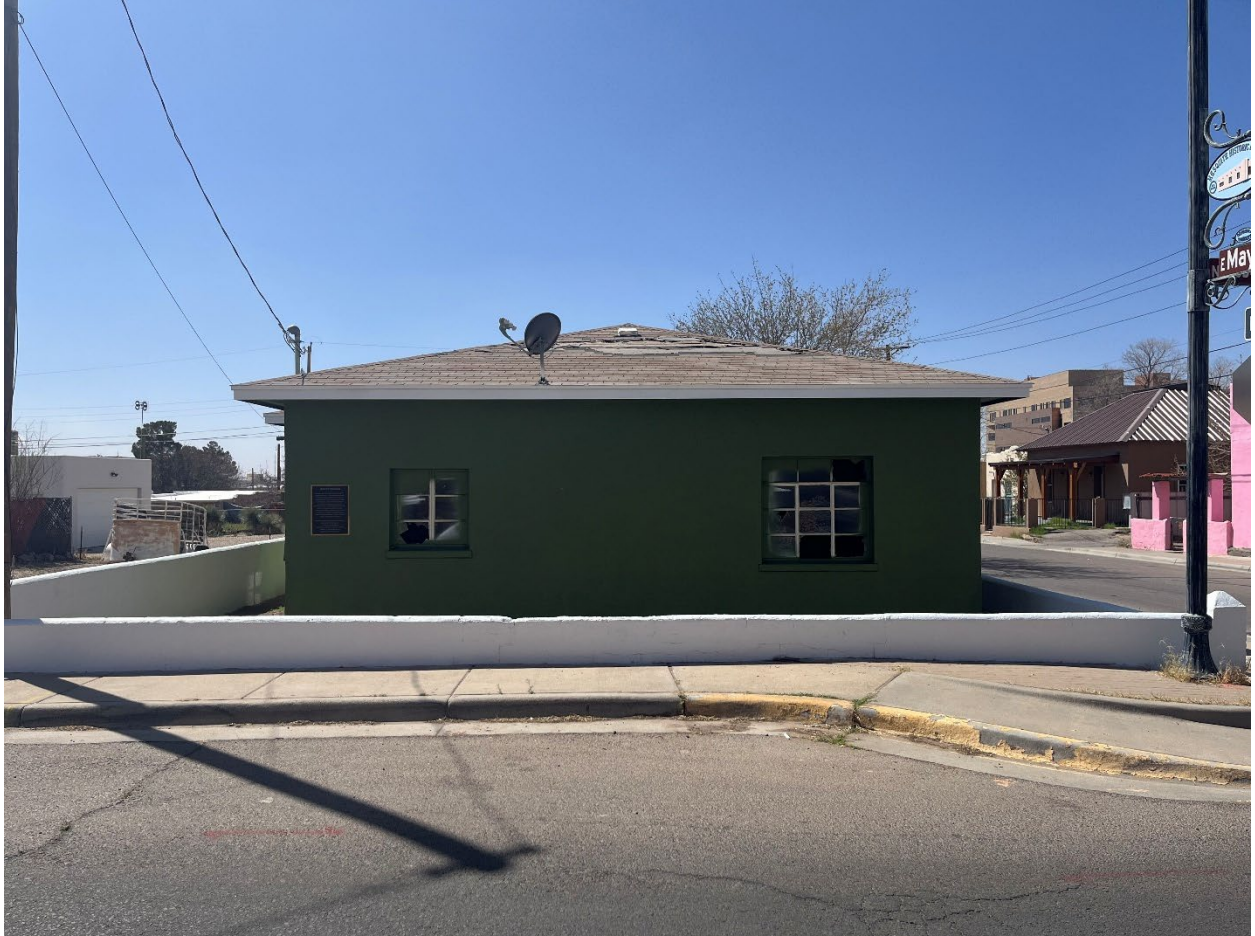
Figure 5: Photo from across Mesquite Street, showing a prominent facade with mural plaque.
