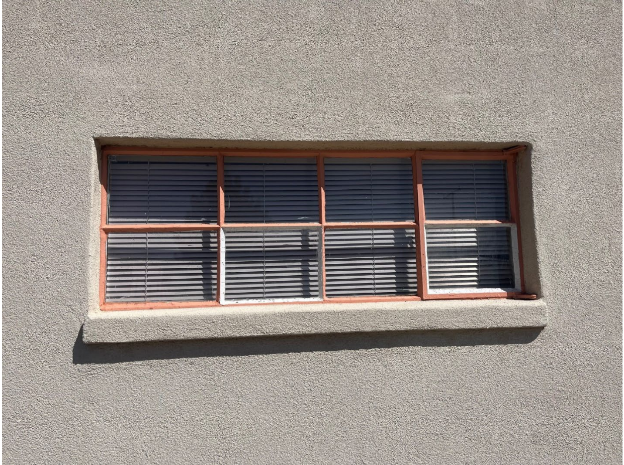
Figure 10: Example of a repaired metal casement window at neighboring 2630 San Andres Drive, across the street from 440 E. May.
