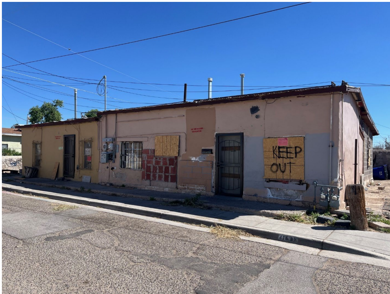
Figure 7: Main façade of the duplex on Lucero Avenue.
