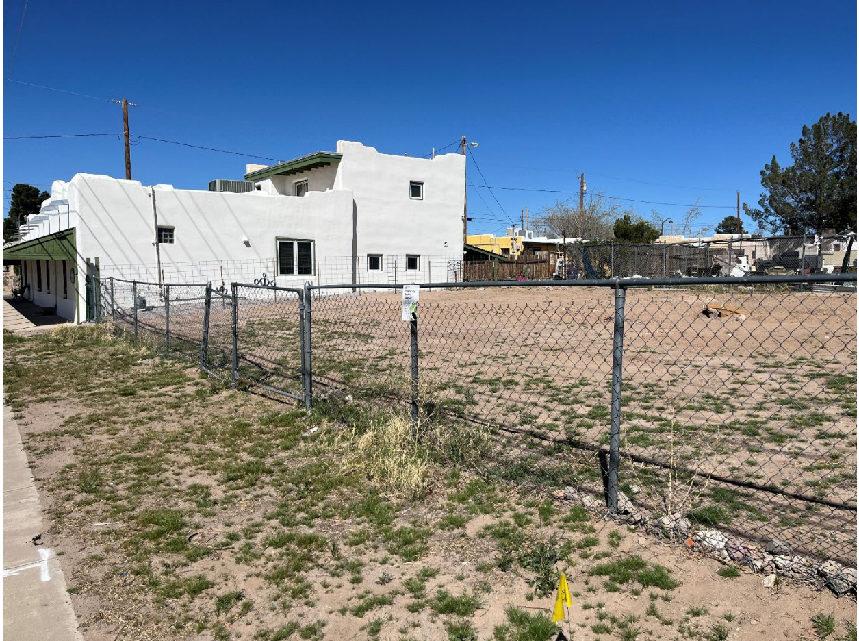
Figure 3: Photo across property, showing south façade of 640 N. Mesquite, camera facing northeast.
