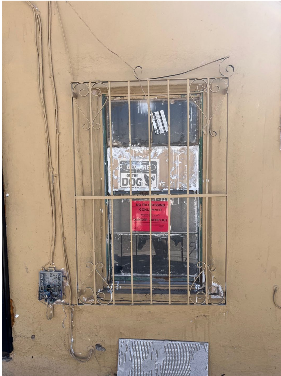
Figure 10: Window on east unit of the duplex on Lucero Avenue.
