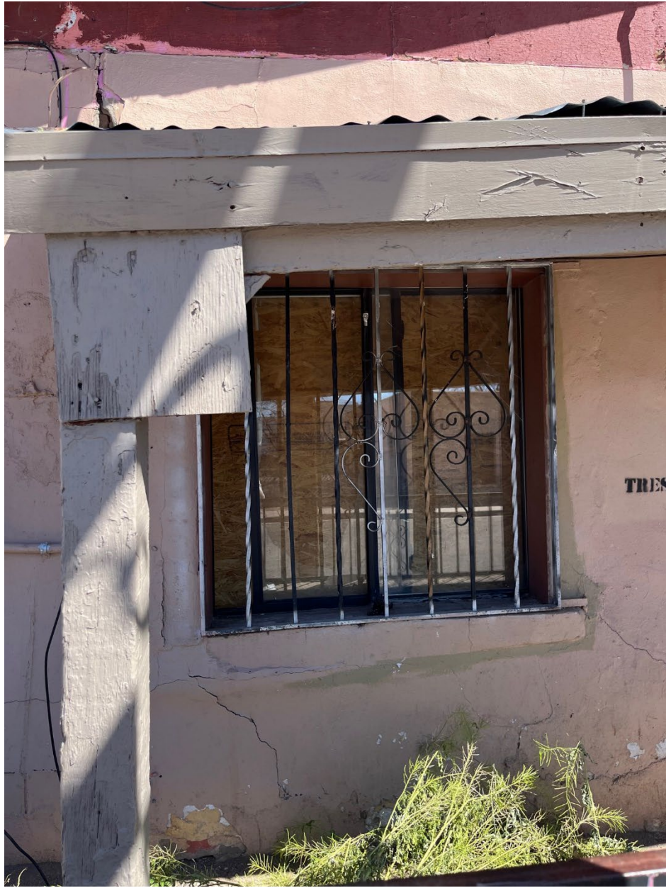
Figure 5: North window on main façade of the house fronting San Pedro Street.
