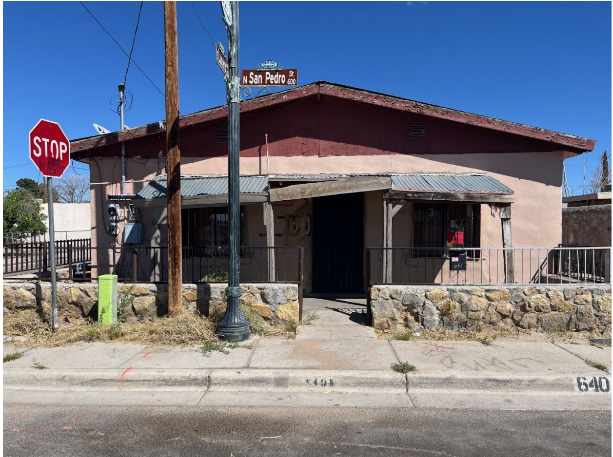
Figure 3: Photo of main façade of the house fronting San Pedro Street, taken from the middle of San Pedro Street.
