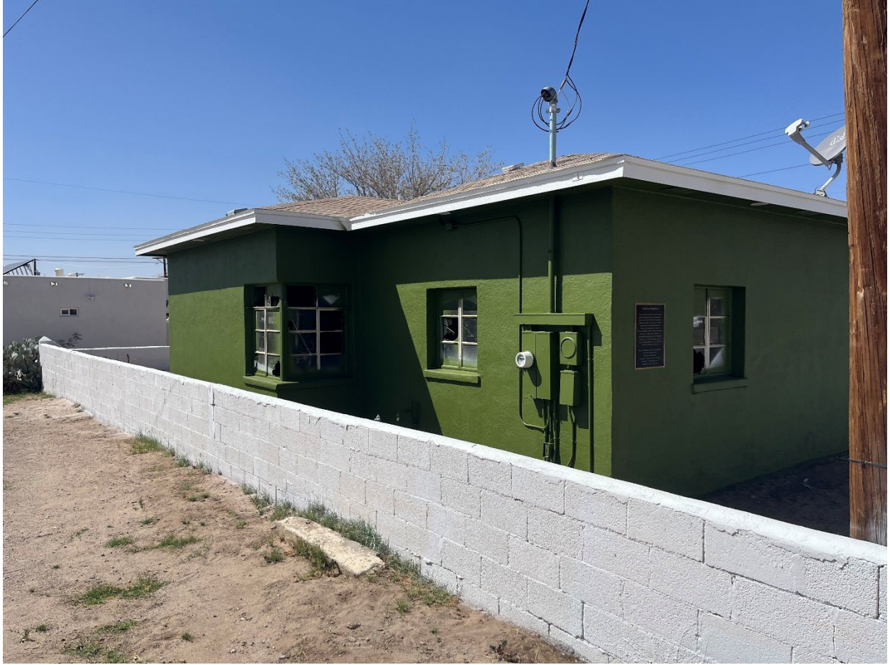
Figure 7: Image of the rear of the property, taken from the sidewalk on Mesquite Street.
