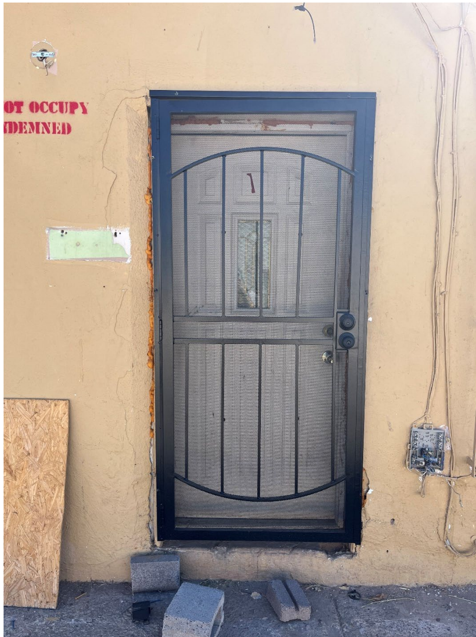
Figure 11: Door on east unit of the duplex on Lucero Avenue.
