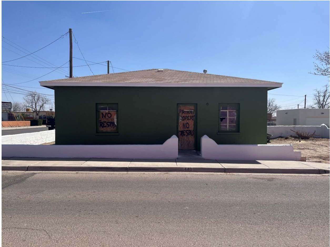
Figure 4: Photo of front facade of building from across May Avenue.
