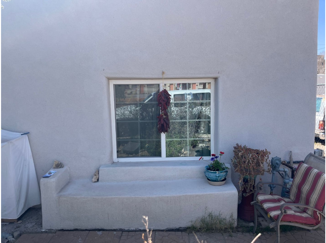
Figure 9: Example of fake-muntin vinyl slider window on the front façade of 216 S. Mesquite.
