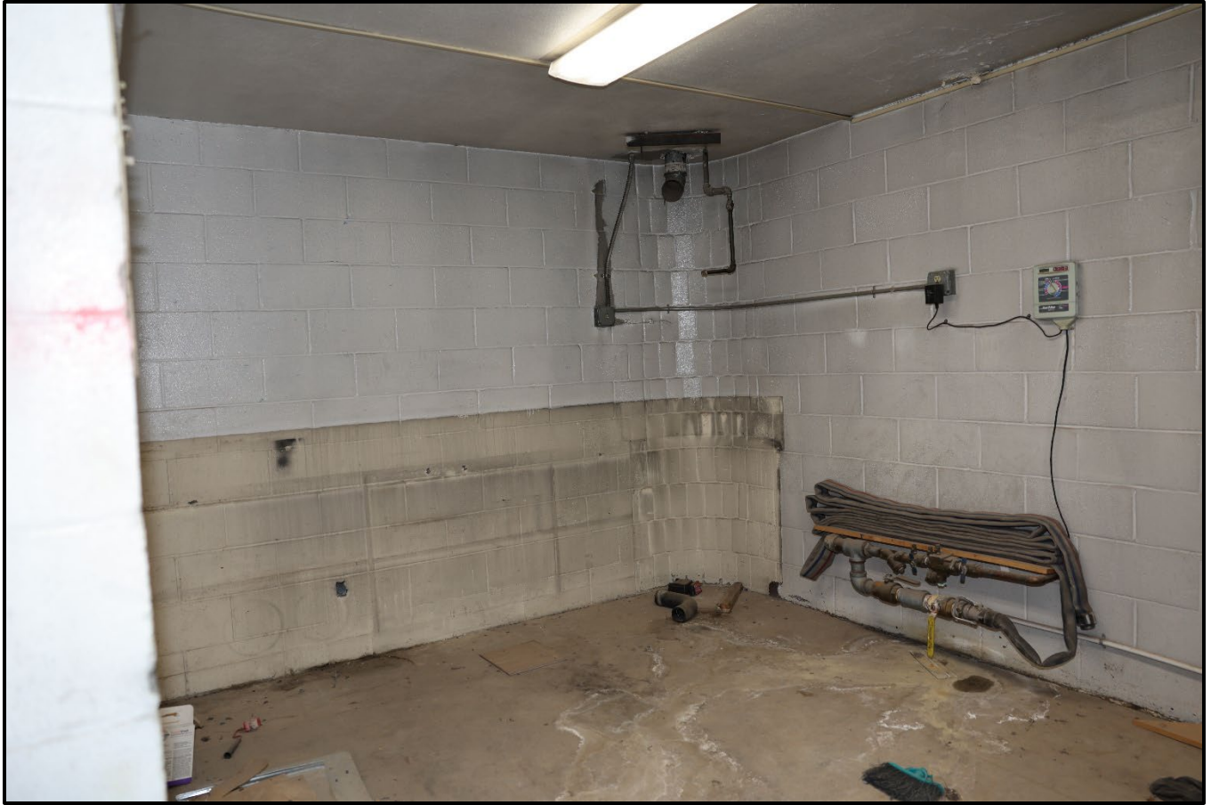
Figure 20: Photo of the interior of the work room, attached to the engine bay/apparatus room to the north.
