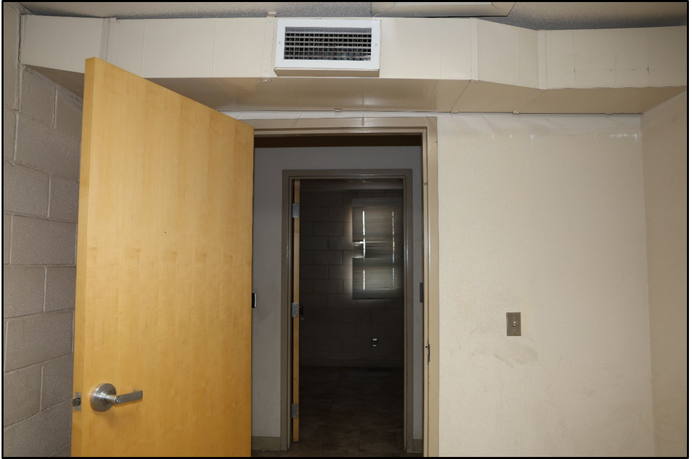
Figure 37: Photo from the interior of the bunkroom, looking into the hallway with another bunk room in the background.
