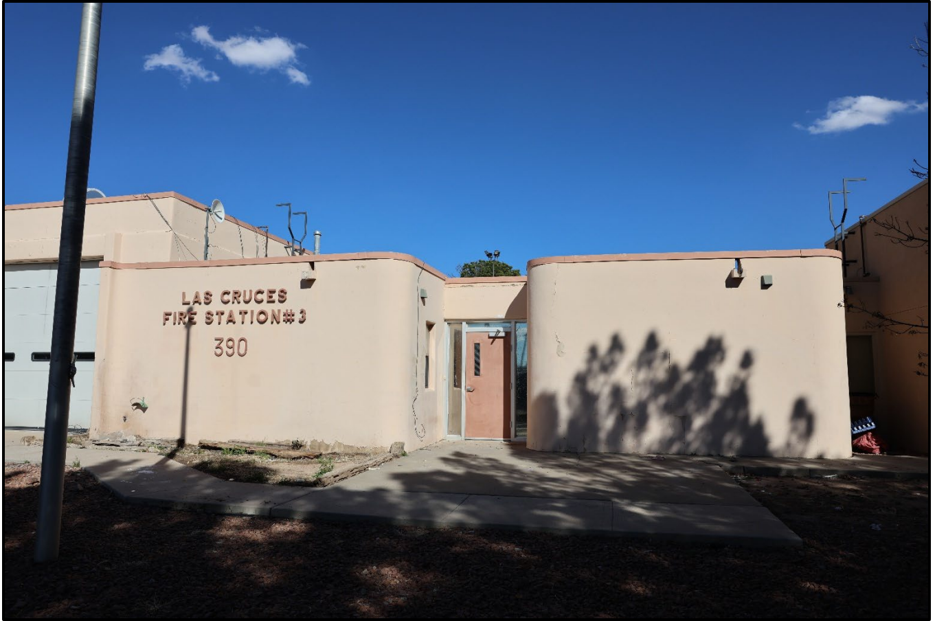
Figure 16: Photo of the main entrance to the station, taken from the west.
