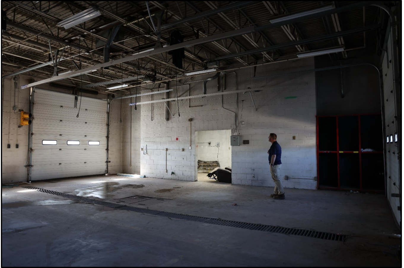
Figure 19: Photo of the engine bay/apparatus room from the northeast (rear) hallway, looking northwest.
