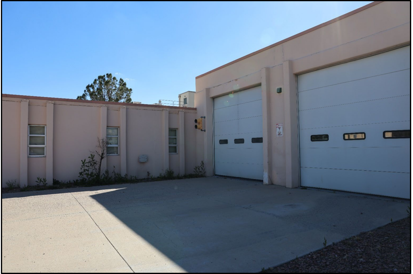
Figure 12: Exterior of the bunk room wing, where it connects with the east entrance (non-emergency) to the engine bay/apparatus room. Bay doors are replacements.
