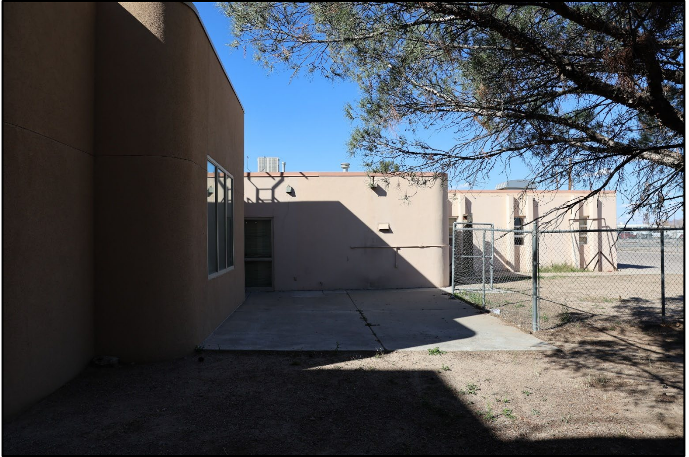
Figure 9: Photo of the south facade of the building, capturing the original design of the kitchen and the bunk room wing, taken from the southern edge of the property.
