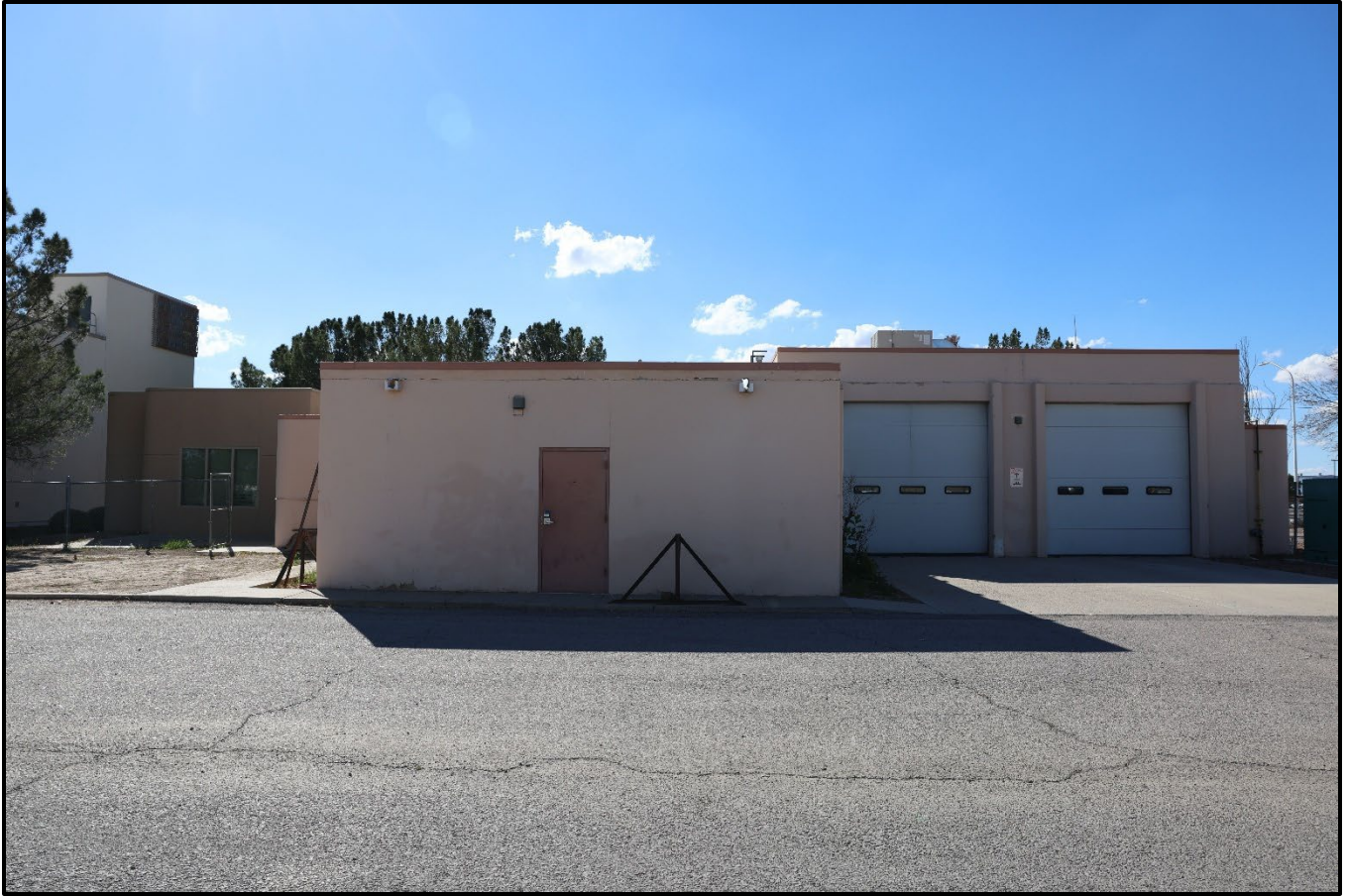
Figure 11: East facade (rear) of the building, taken from the access road to the rear of the current Fire Station No. 3 (380 N. Valley Drive).
