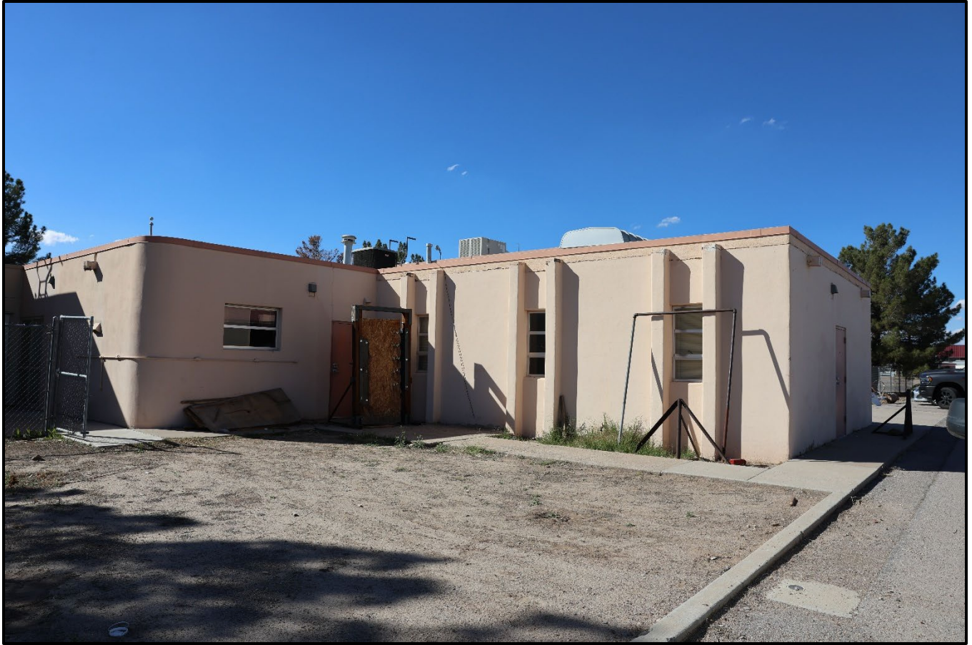
Figure 10: Photo of the bunk room exterior where it meets the main body of the building (kitchen), taken from the southeastern corner of the property.
