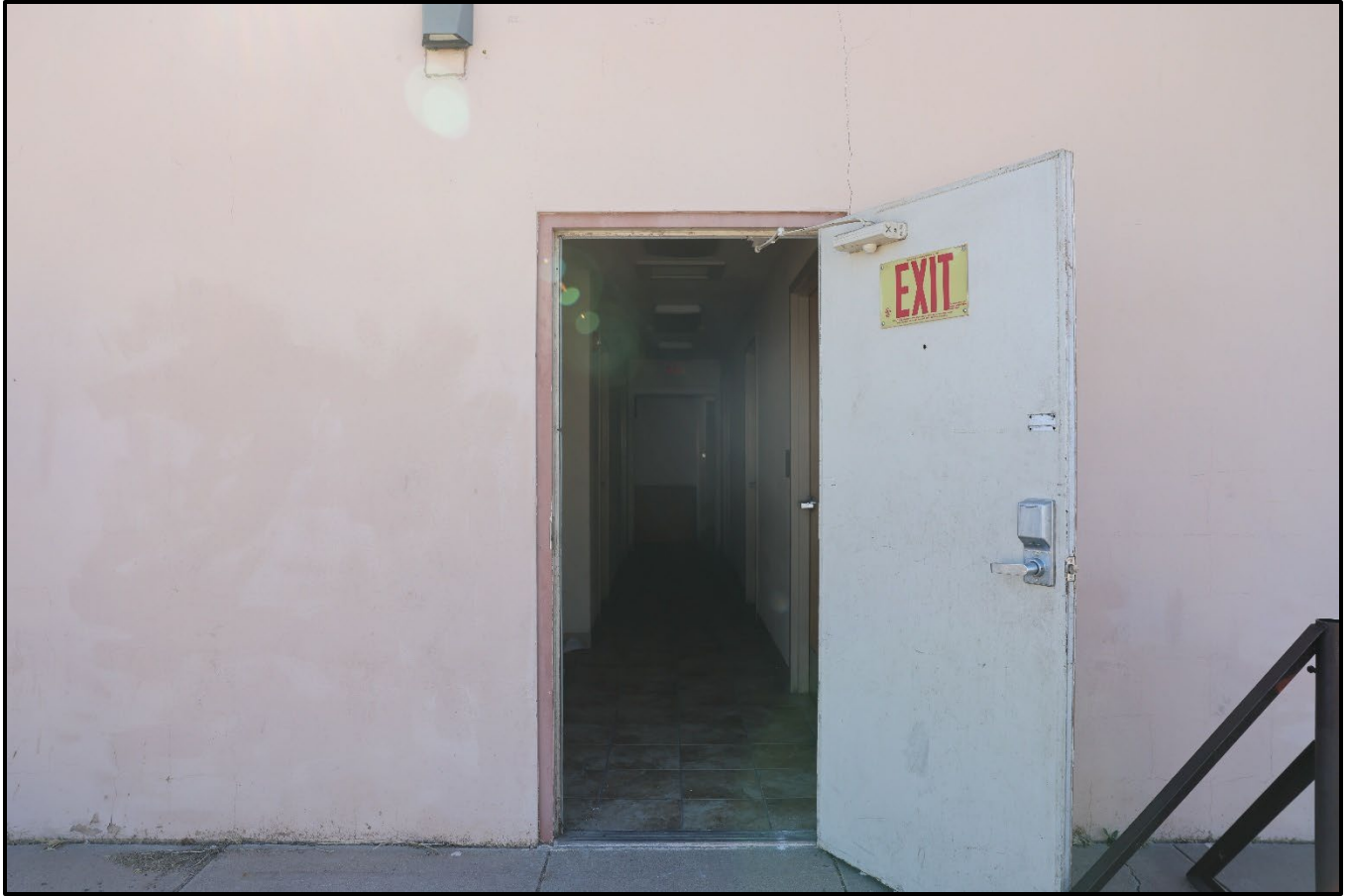
Figure 17: Photo of private entrance to the bunk room wing (east facade), taken from the east.
