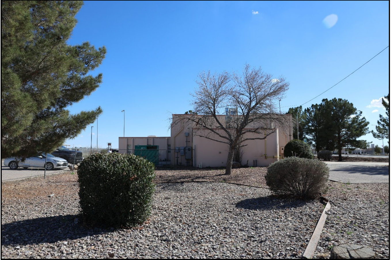
Figure 13: North façade of building, taken from the curb along the northern property line.
