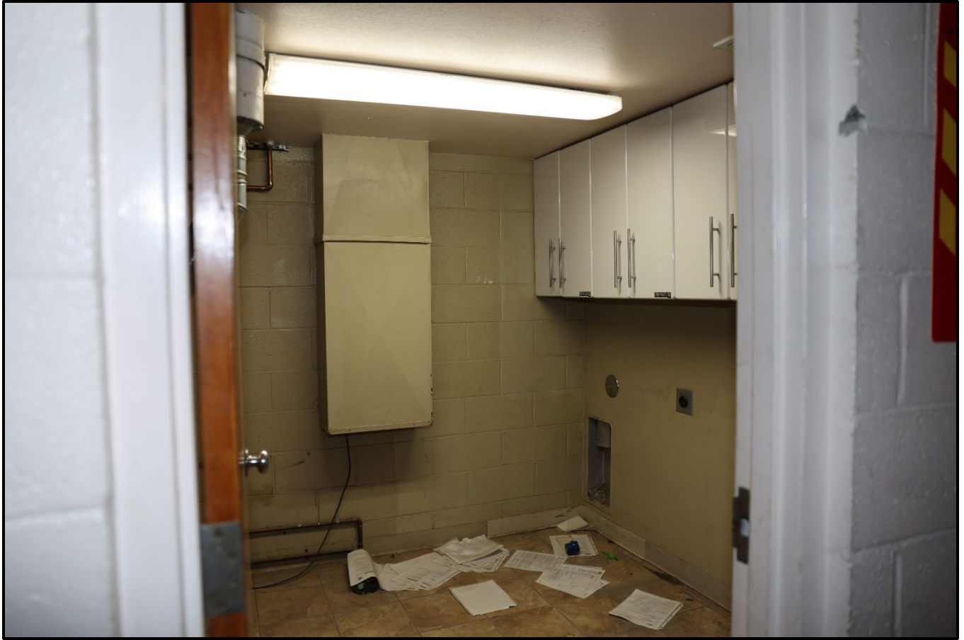
Figure 33: Interior of utility room, looking northwest.
