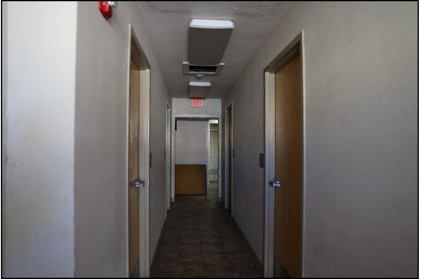
Figure 18: Photo of the bunk room hallway from the threshold, looking east.
