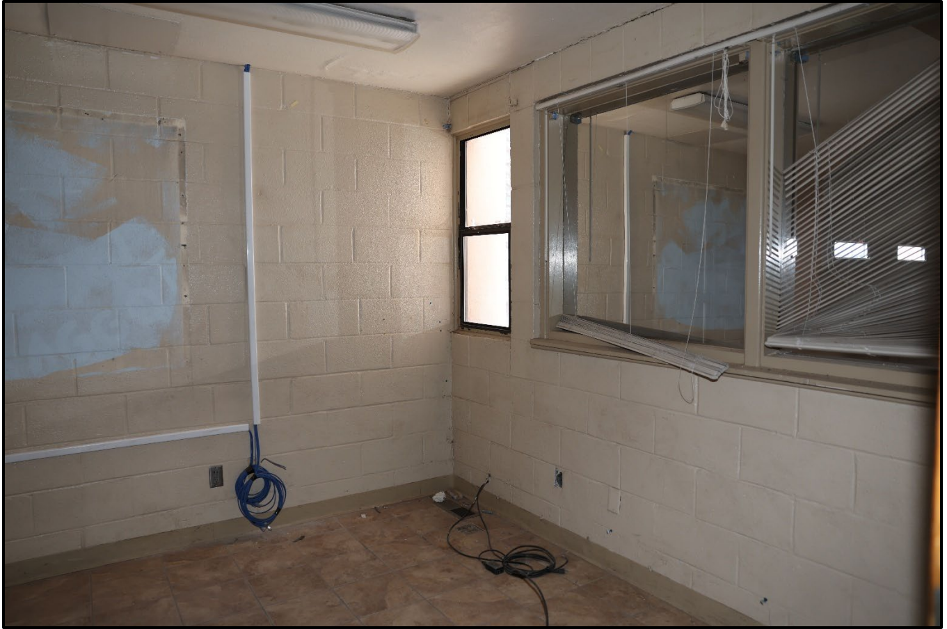
Figure 24: Photo of the interior of the duty room, on the western-most side of the building. Note windows looking into the engine bay/apparatus room.
