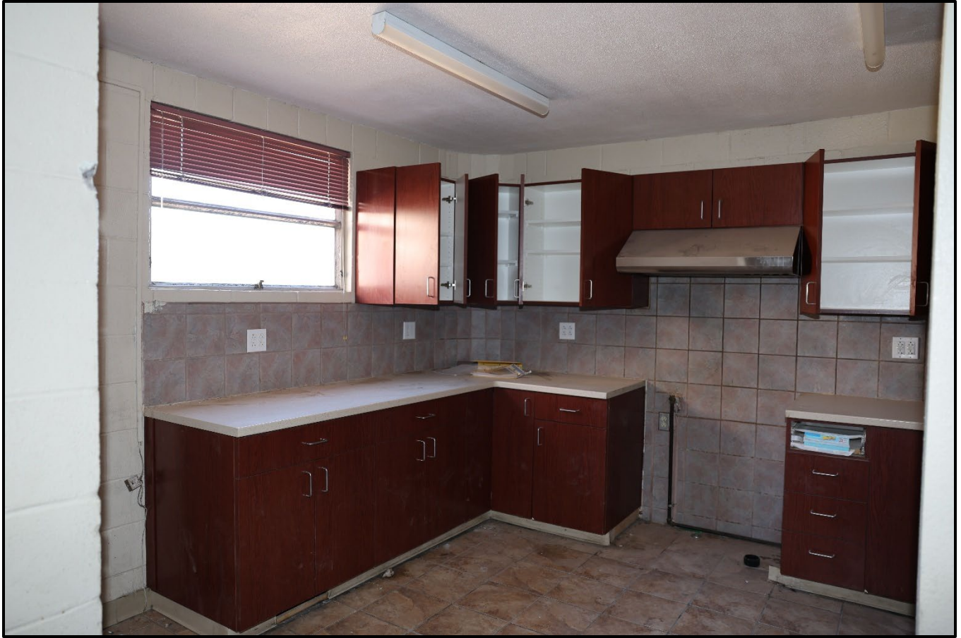
Figure 31: Interior of the kitchen (altered), taken from the northwest looking southeast.
