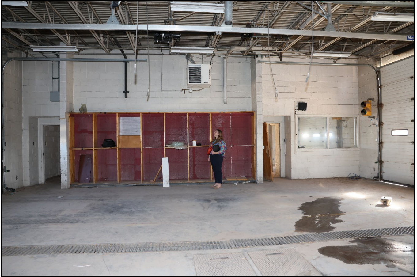
Figure 22: Photo of the engine bay/apparatus room looking south. Note the east and west hallway access doors.
