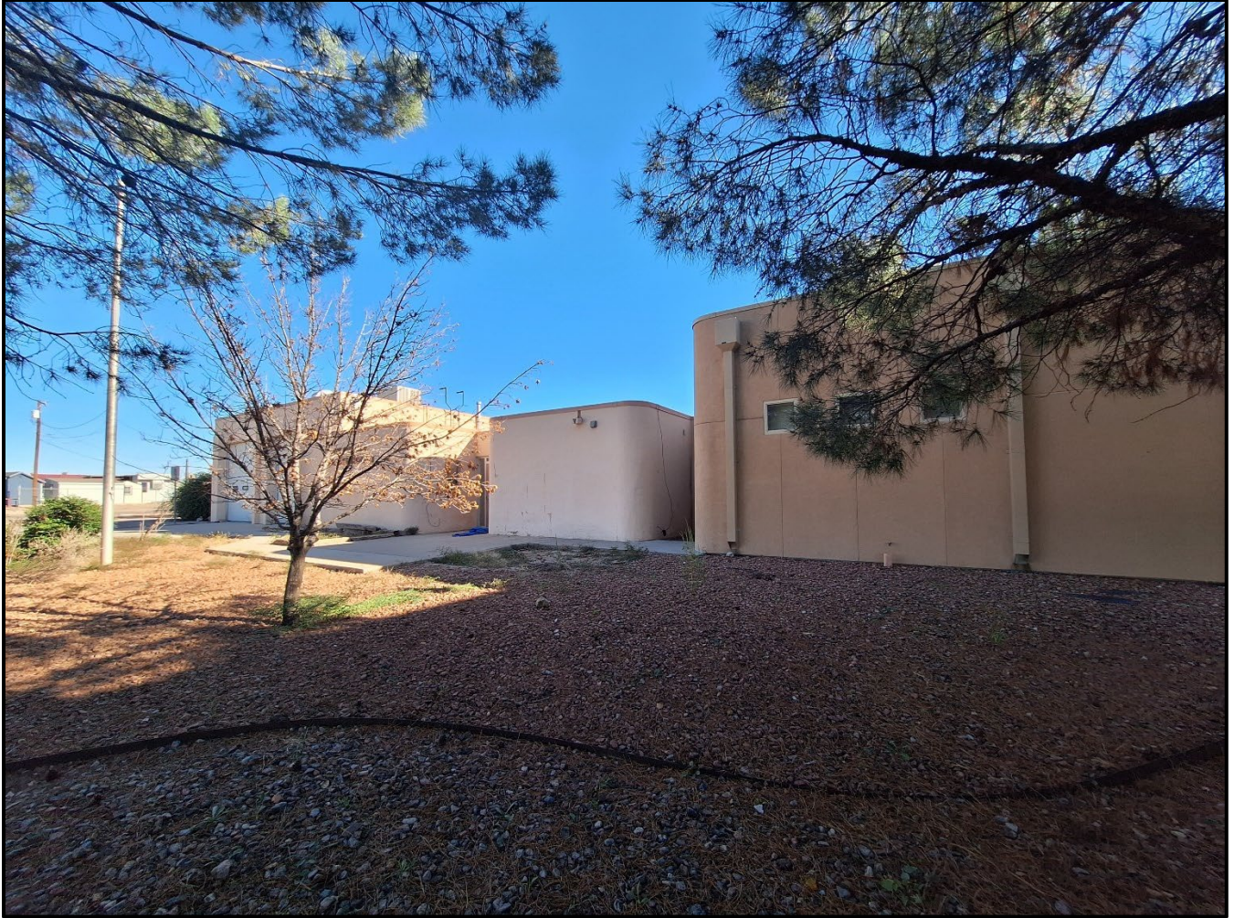
Figure 8: Photo of the west facade, taken from the southwest beneath two trees. Photo taken October 29, 2025, by Raymond Burchfield.
