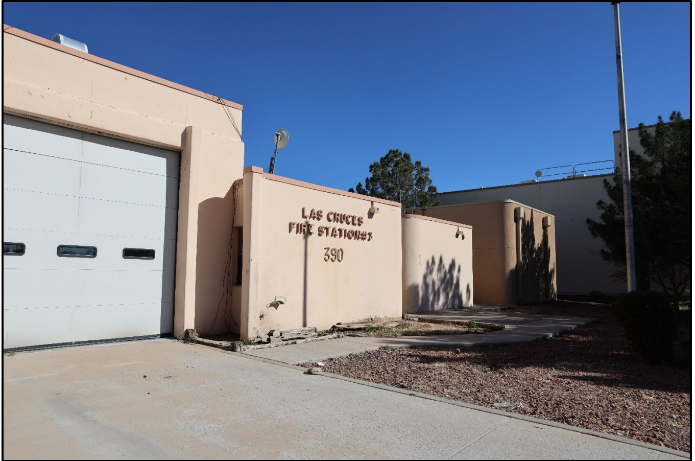
Figure 15: Photo of the main entrance to the fire station, located on the west facade, taken from the northwest access drive and the engine bay/apparatus room (exit).
