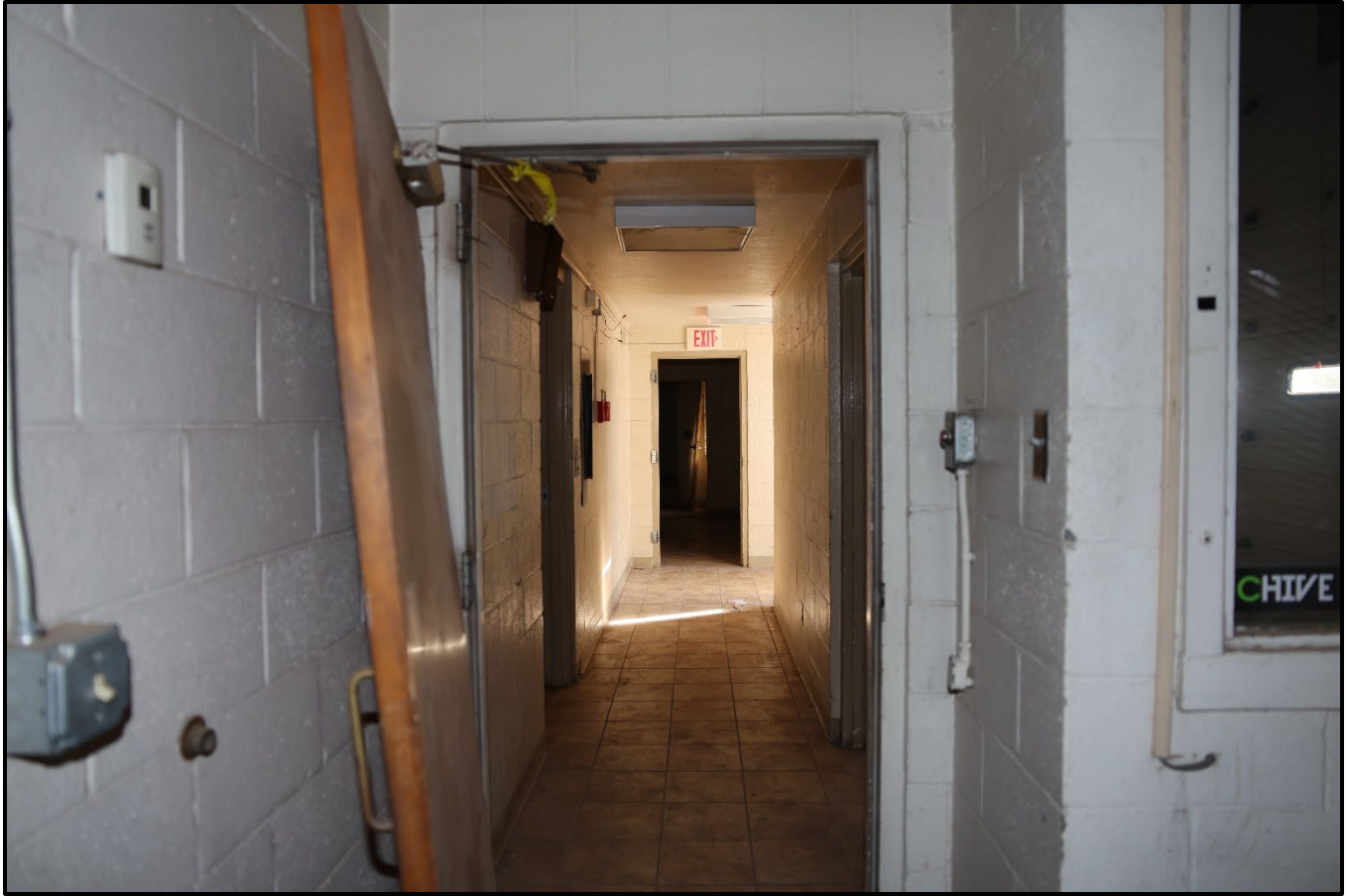
Figure 23: Photo of the west hallway access, looking south towards the gym addition.
