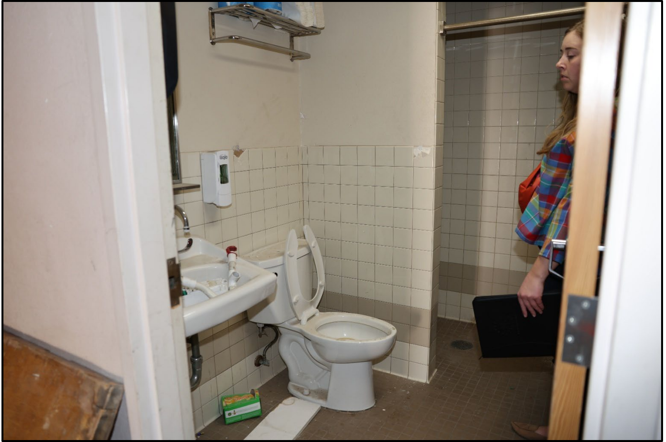
Figure 34: Interior of the shared bathroom adjacent to bunk room wing, looking southwest.
