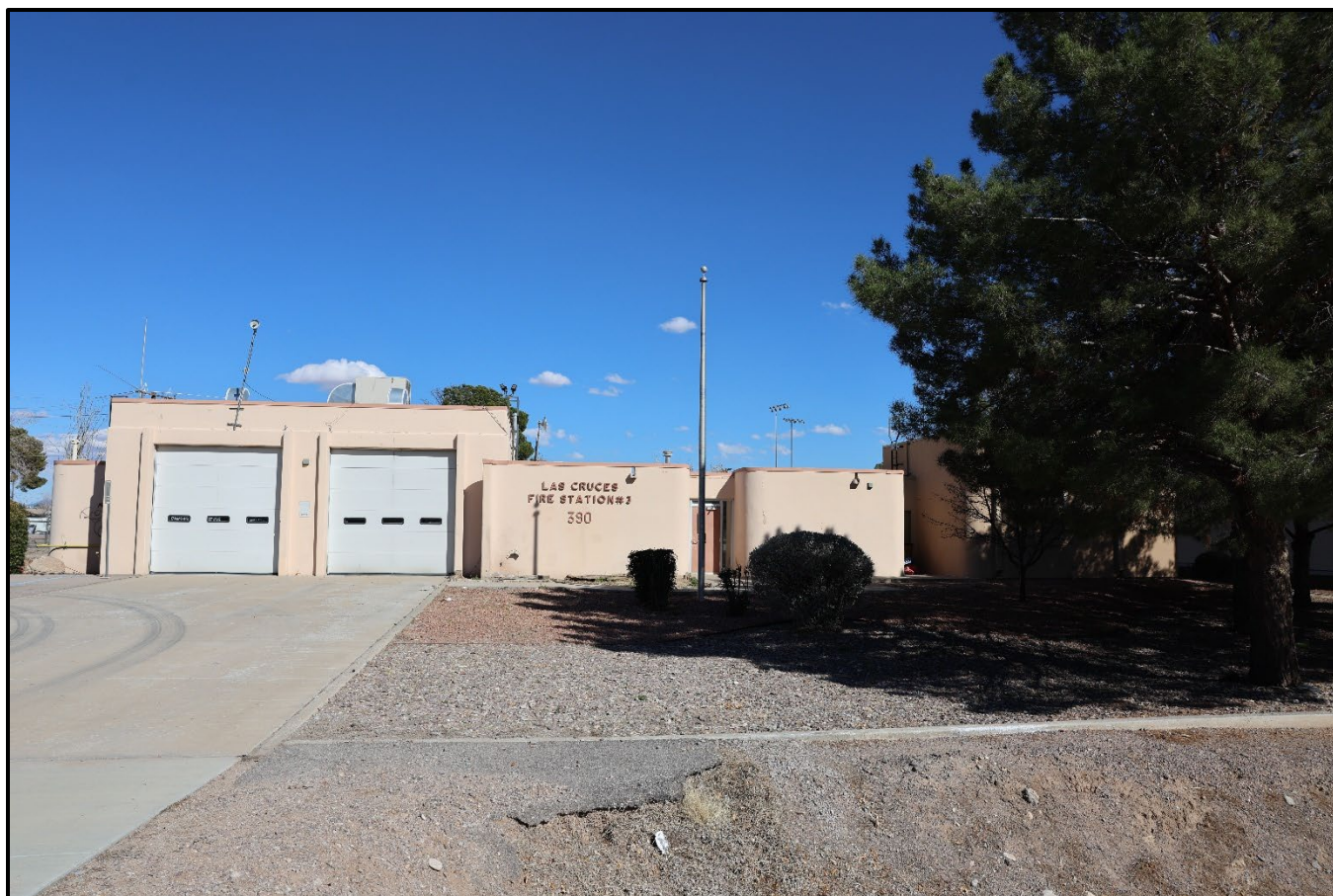
Figure 6: West facade (main) of Fire Station No. 3, taken from the sidewalk.
