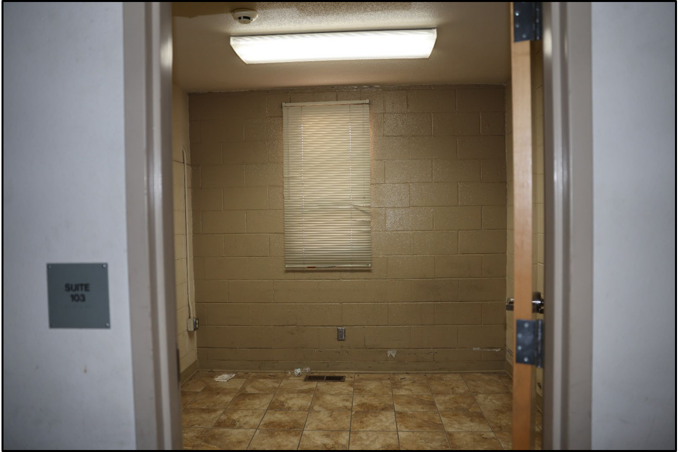
Figure 36: Interior of a bunk room, from the threshold.
