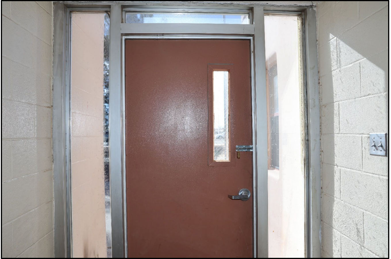
Figure 26: Interior of main entrance (west facade), looking west.
