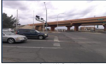
Corner 1 No Ramp (12)
