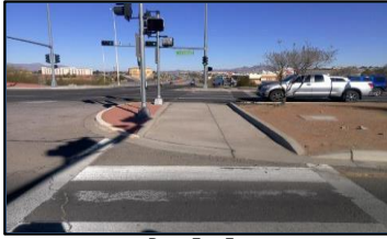
Ramp East F
