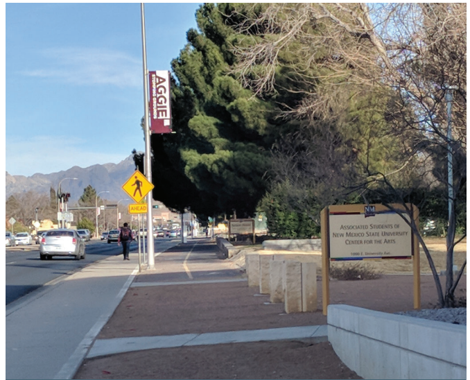
The end of the two-way separated bike lane on University Avenue
