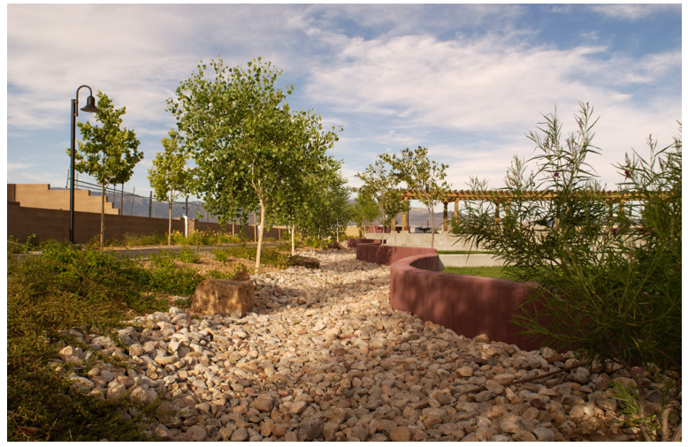
Low Impact development feature, bioswale
