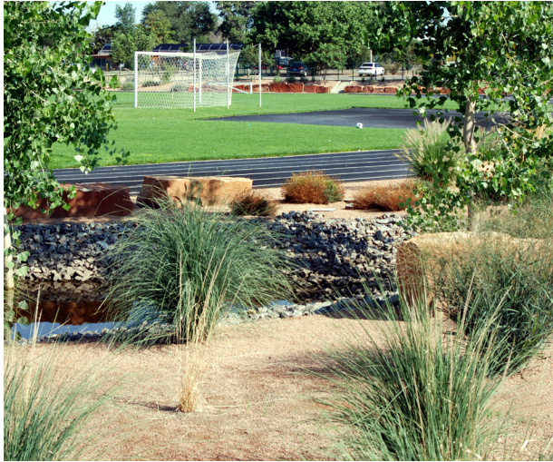
Low Impact development feature, bioswale
