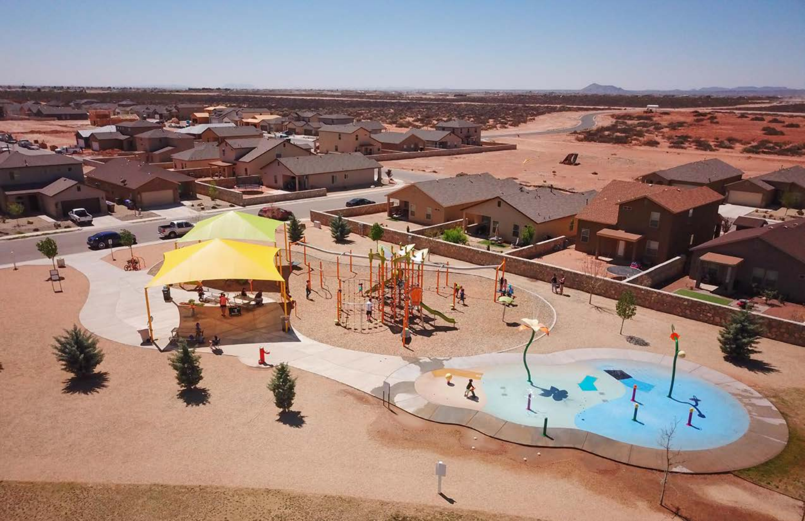
The scenario planning process considers the development status of new subdivisions such as Metro Verde (above), including the status of “entitled” lots which may be platted but do not yet contain homes or other buildings
