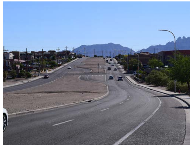
Lohman Avenue (above) is a major arterial roadway with right-of-way characteristics that can accommodate the addition of future travel lanes in anticipation of higher traffic volumes.
