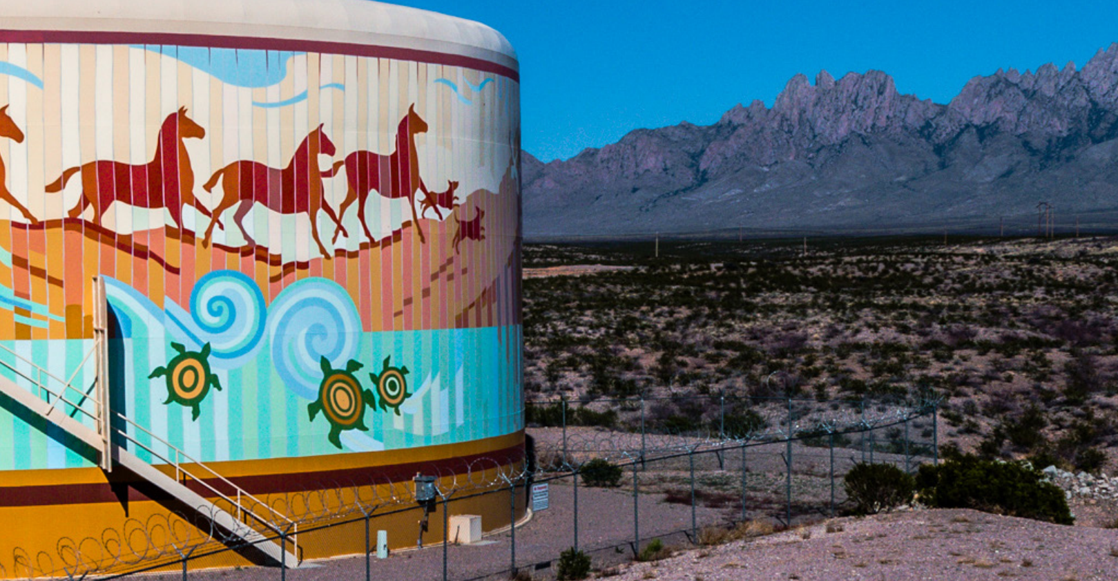
Water storage tanks (above) serve a necessary, utilitarian purpose, and in Las Cruces serve as an opportunity to showcase artistic abilities as well.
