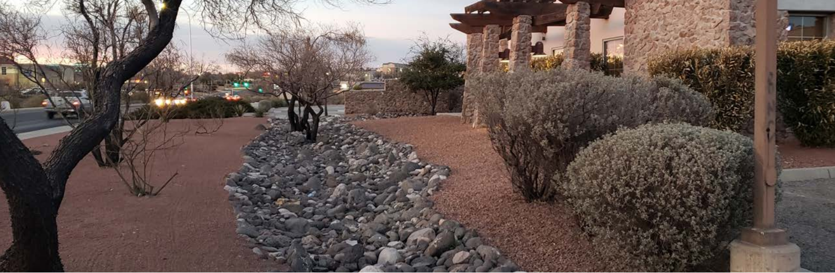
Reducing the amount of impervious surface in new developments (above) has helped reduce and manage stormwater run-off.
