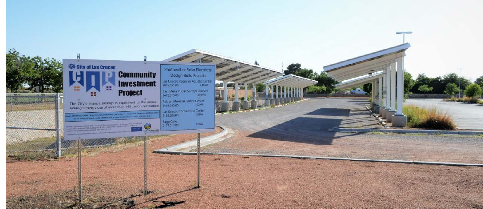
The City of Las Cruces has invested in solar panels at many municipal facilities to generate energy (below).
