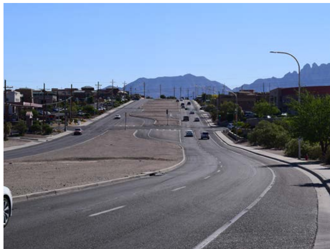
Lohman Avenue (above) is a major arterial roadway with right-of-way characteristics that can accommodate the addition of future travel lanes in anticipation of higher traffic volumes.
