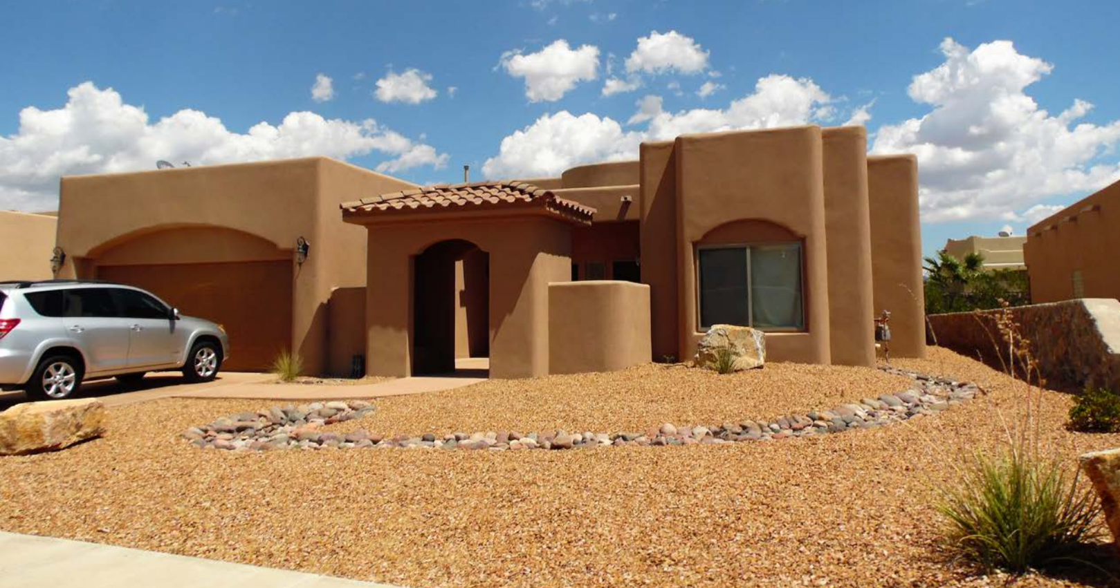
Many new developments in Las Cruces utilize building materials, forms, colors, and styles that are complimentary to the region's natural and cultural heritage.
