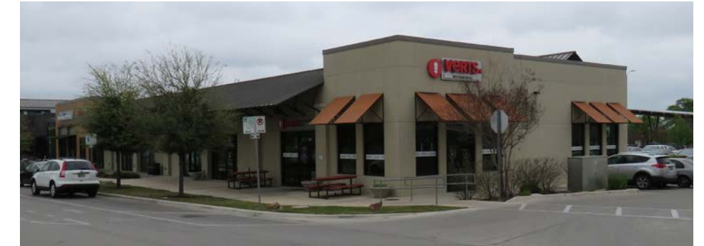
Neighborhood Centers may include single-story and single-use buildings but should be easily accessible to surrounding residents and arranged in a manner that supports and entices pedestrian activity within the roadside.
