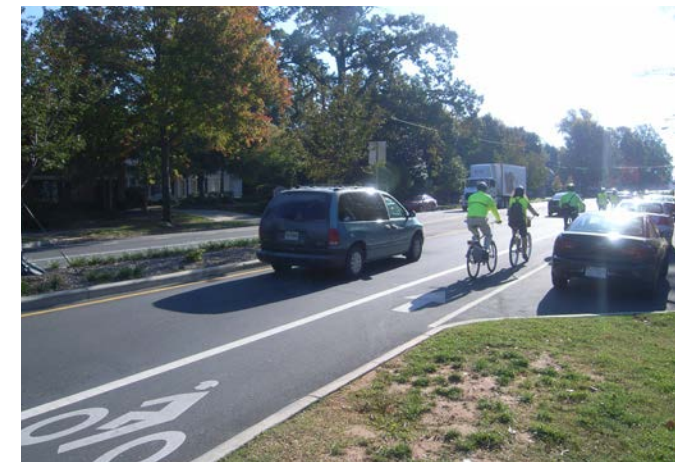
Urban streets can be candidates for lane reductions. The roadway above was converted from a four-lane minor arterial street into a three-lane avenue with on-street parking, bicycle lanes, and intermittent medians (above).
