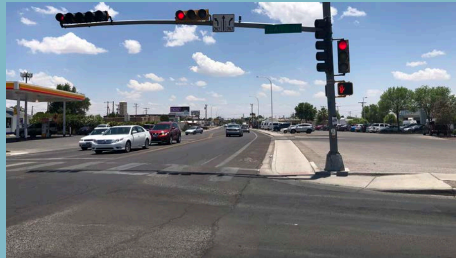
S. Solano Drive at Idaho Avenue (above).
