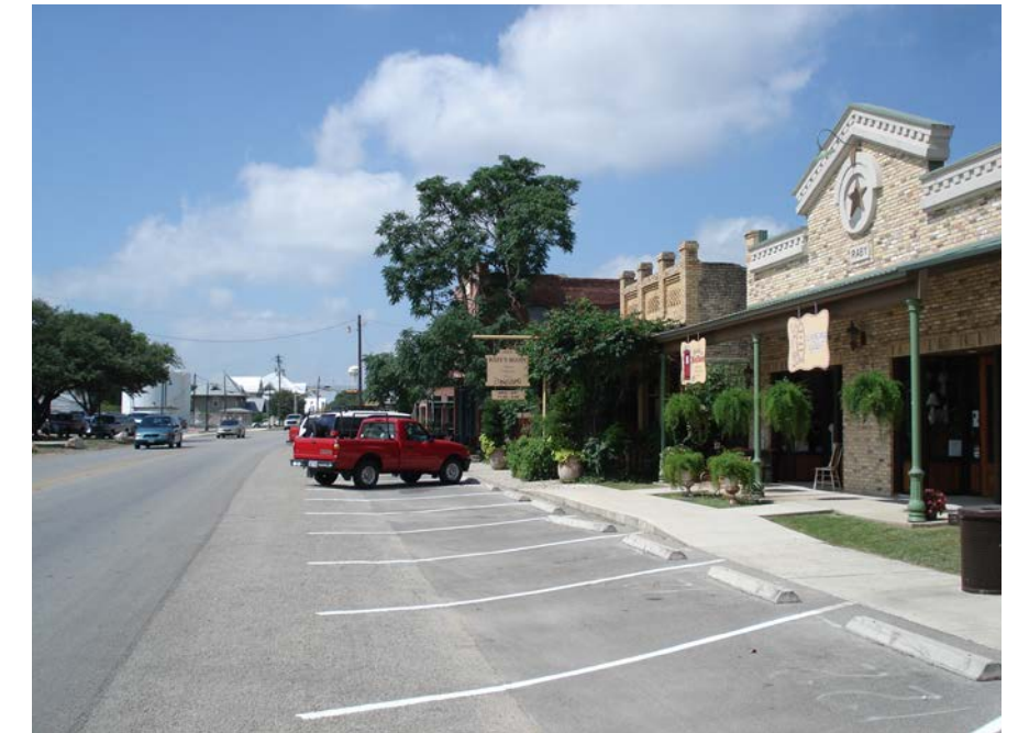
The retrofitted street above includes a new lane of on-street parking and active roadside elements. The street was constructed with public funds while adjacent infill buildings conformed to form-based zoning provisions.
