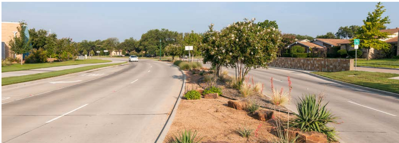
Suburban streets may have medians (above) as a method of access management, and to create a consistent community character.
