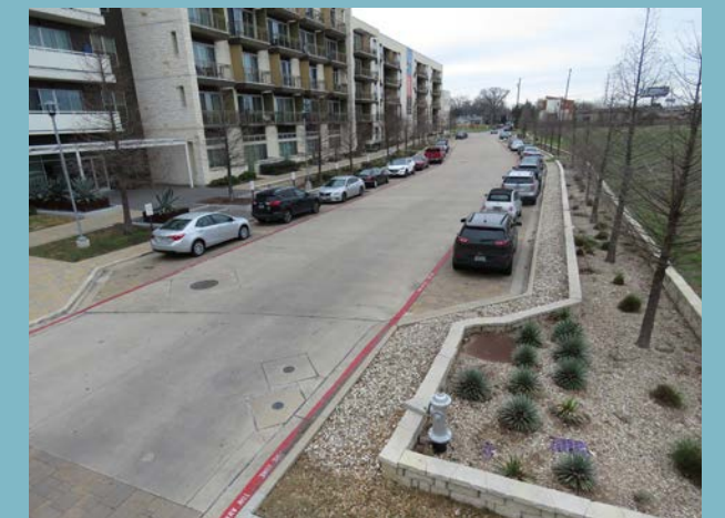
Green streets integrate low-impact stormwater management principles such as permeable pavement and bioretention planters (above).
