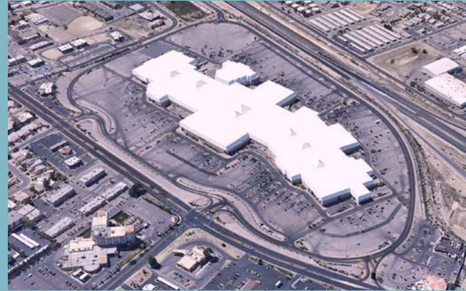
Existing Mesilla Valley Mall (above).
