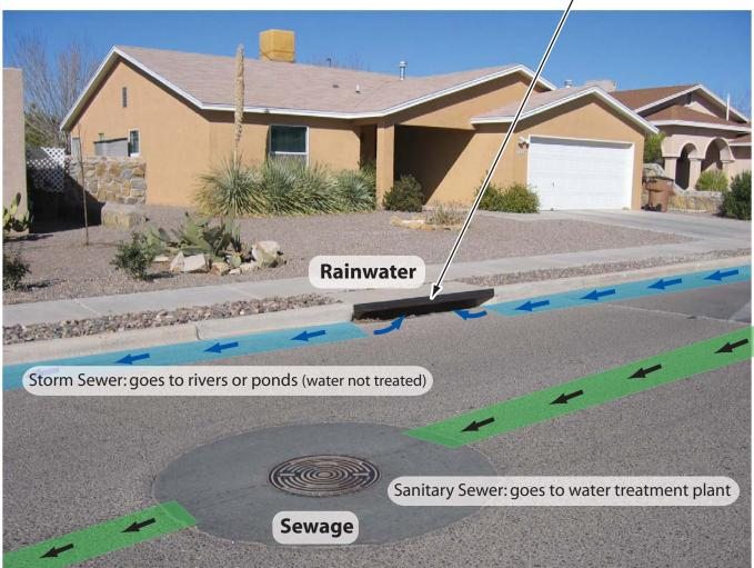
The "sanitary sewer" system is designed to carry sewage from homes and businesses to a water treatment plant. After the sewage is treated, the water can be reused/reclaimed for industrial purposes and agricultural irrigation.
