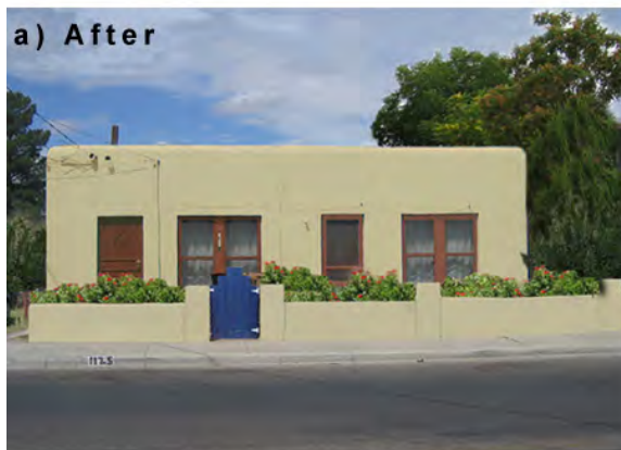
Facade enhancements shown above include new paint on the house & wall, a new gate, and new trees & shrubs
