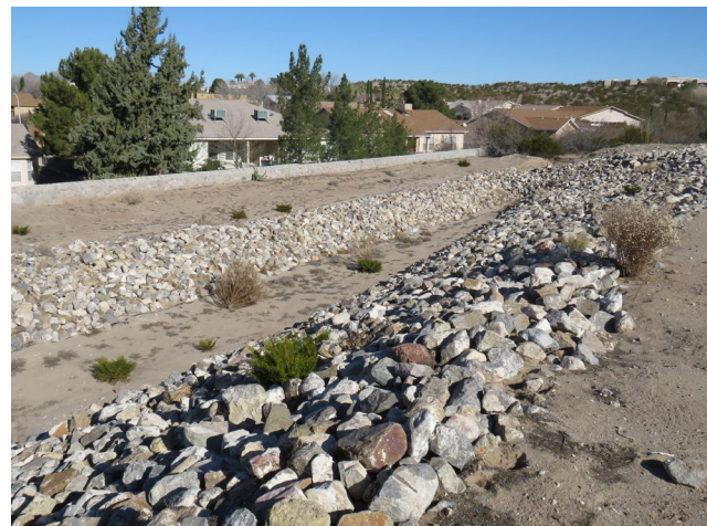
Arroyos represent natural pathways for storm water drainage, but may also be improved to accommodate increased runoff and seasonal recreational activities.
