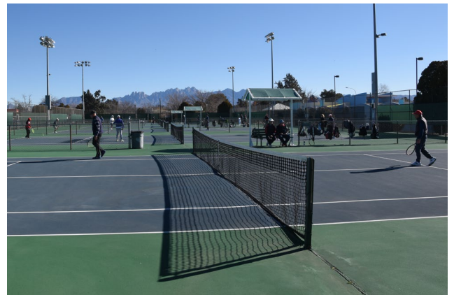
Lions Park West tennis court complex. Sport court surface quality is fairly high.
