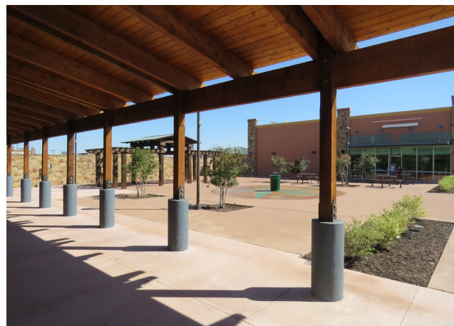
Social space incorporated in a commercial shopping plaza. Future tenants can utilize the space for outdoor seating and performances.
