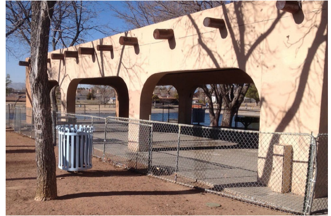
R.L Young Park pavilion and event rental space is currently inaccessible.
