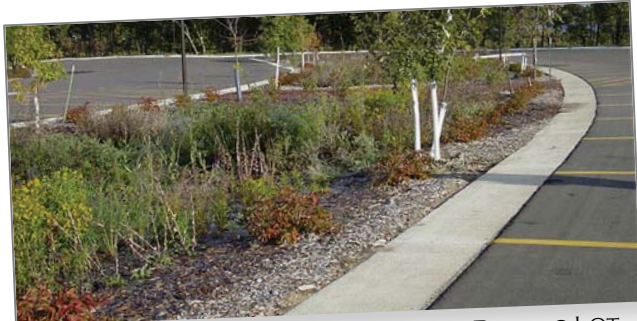
GREEN INFRASTRUCTURE: BIOSWALE IN PARKING LOT
