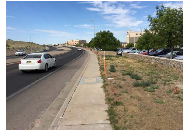
Current conditions: East Lohman Avenue Source: Sites Southwest
