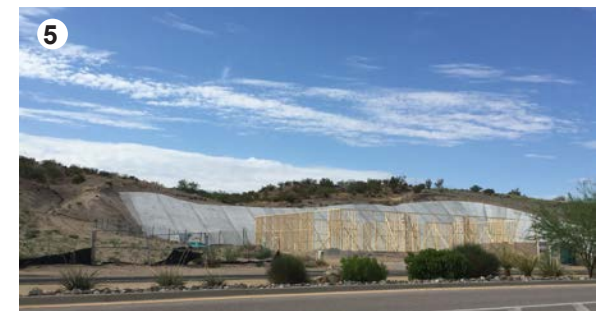
New commercial development along East Lohman Ave illustrates the steep slopes of the undeveloped hillside in the planning area.
