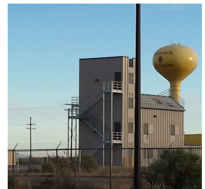
City Fire training tower adjacent to the fire station.
