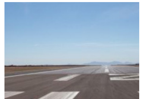
Approach to Runway 12. Image by Delta Airport Consultants
