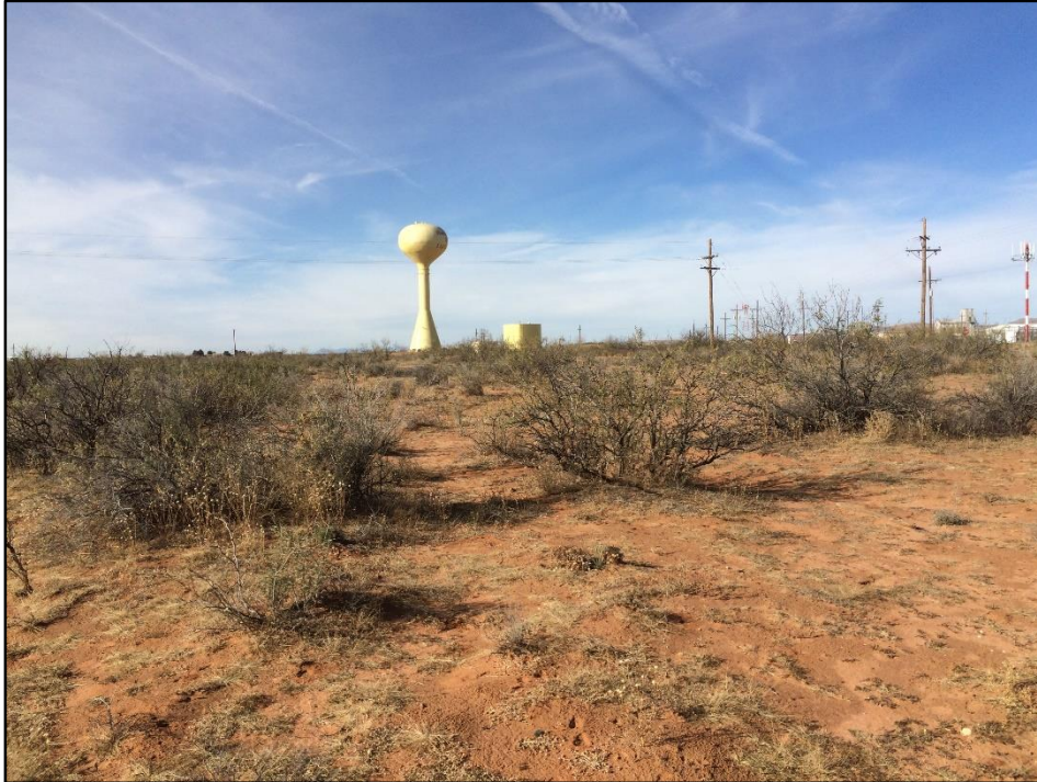
Photo 1. Facing west in southern project area, south of terminal building.
