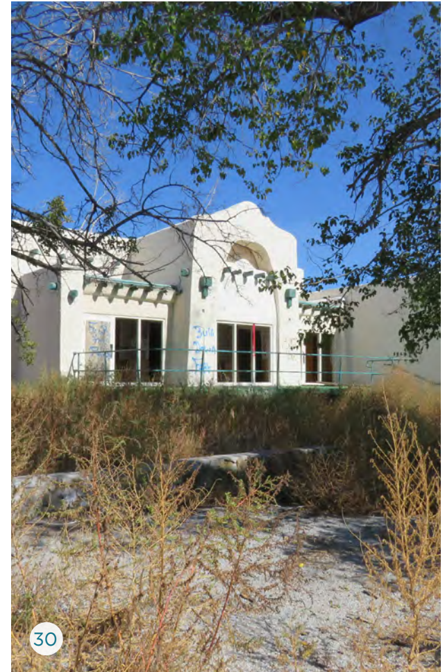
IMAGE 30: The Las Cruces Country Club clubhouse building was designed by Henry C. Trost - an architect of regional significance. Incorporating the structure into future development scenarios provides a link to the site’s past.
