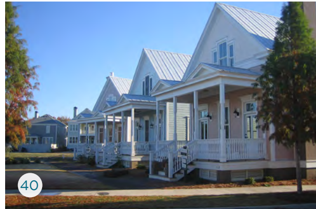
IMAGES 40 & 41: Garden homes and townhouses are among the many housing types that may be incorporated into Focus Area A character areas.
