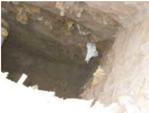
Photo #3 Test pit 4, debris.
