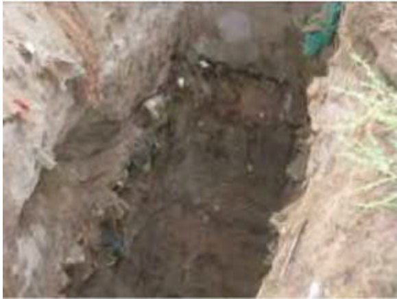
Photo #7 Test pit 13, debris.
