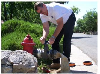
Chris Wilkinson, President of NO-DES and developer of this technology, says, "In essence, we create an above-ground loop in the water distribution system with a portable filtering and disinfection system in the middle. This process results in improved water quality... and conserves two vital natural resources - water, and the energy it took to produce and pump it."
