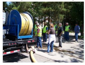
It works like this: a NO-DES truck and 20foot trailer with a massive filtering system pulls up between two fire hydrants in a neighborhood where residents are starting to experience red water.
