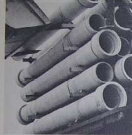
CITY LIFELINES—Another shipment of asbestos-cement water line pipe is unloaded, expanding the life-giving water supply system to new areas.
